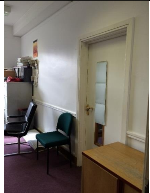
Fig 12: existing right hand side office, with existing doorway to the right and side wall situated between offices.
