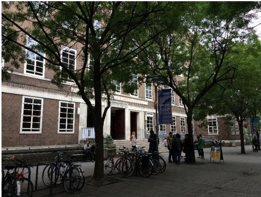
Fig 1: present day, SOAS College Building, southern elevation, author's own.
