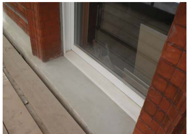
Installed External Cill Detail of Window
