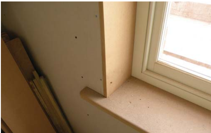
Installed Internal Cill Detail of Window
