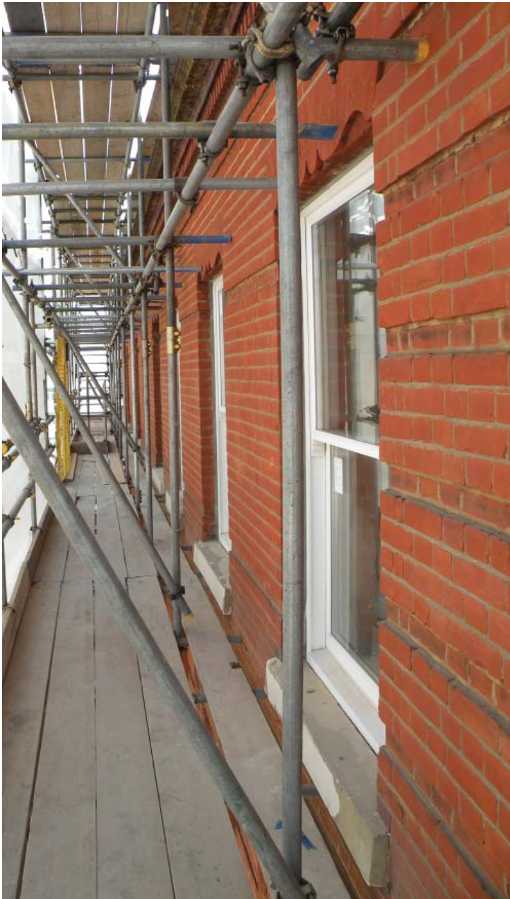
Installed External Detail of Window
