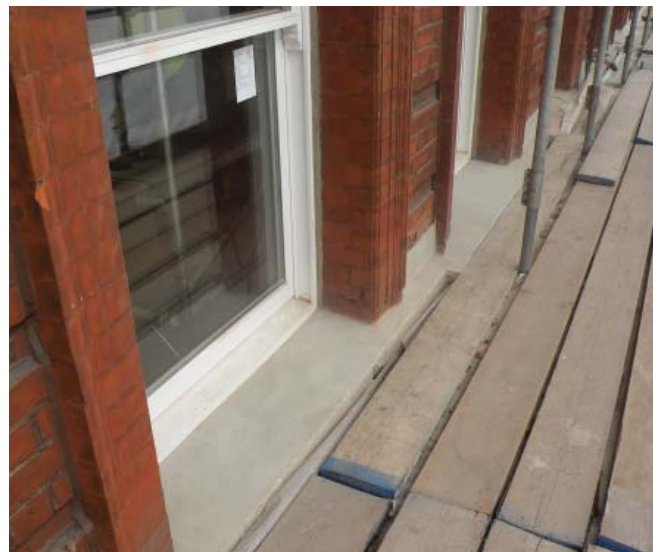
Installed External Detail of Window
