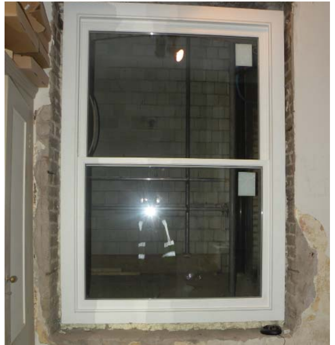
Installed Internal Elevation of Window.
