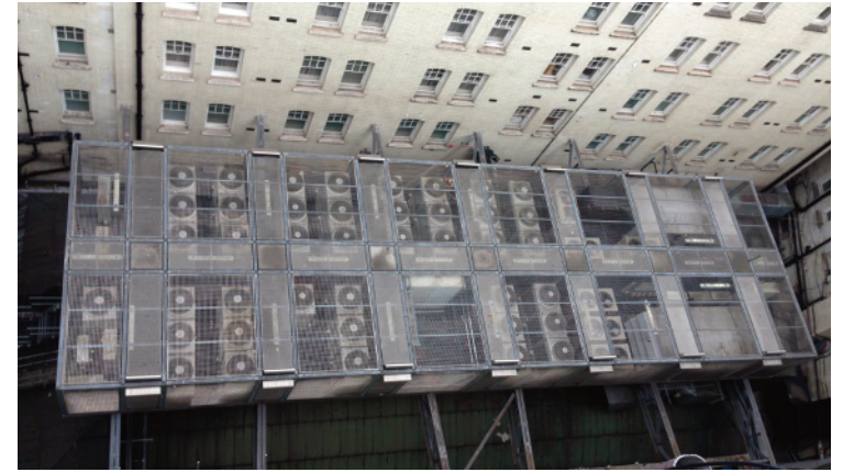
Photo from above (Lantern Roof sits below existing Plant Cage - plant cage also to be cut back to same extent as lantern roof)
