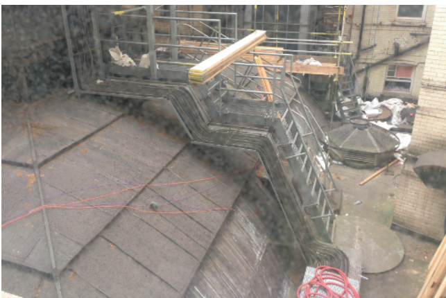
Photos of Existing North-West End of Lantern Roof over Palm Court (showing plant cage above) North-west end to be demolished for creation of External Courtyard - refer drawings for extent
