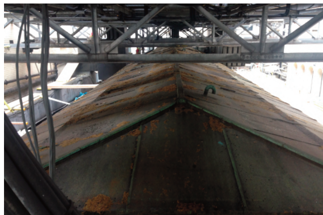
Photos of Existing North-West End of Lantern Roof over Palm Court (showing plant cage above) North-west end to be demolished for creation of External Courtyard - refer drawings for extent
