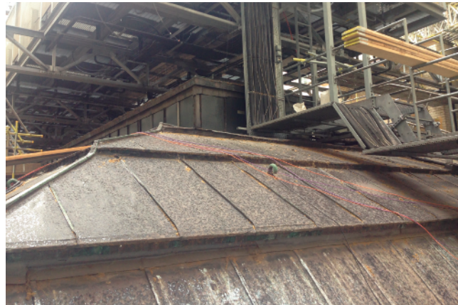
Photo from above (Lantern Roof sits below existing Plant Cage - plant cage also to be cut back to same extent as lantern roof)
