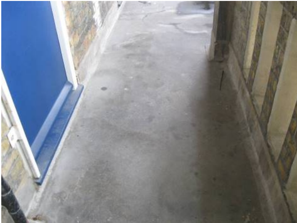
Photograph 25 Access balcony walkway surface
