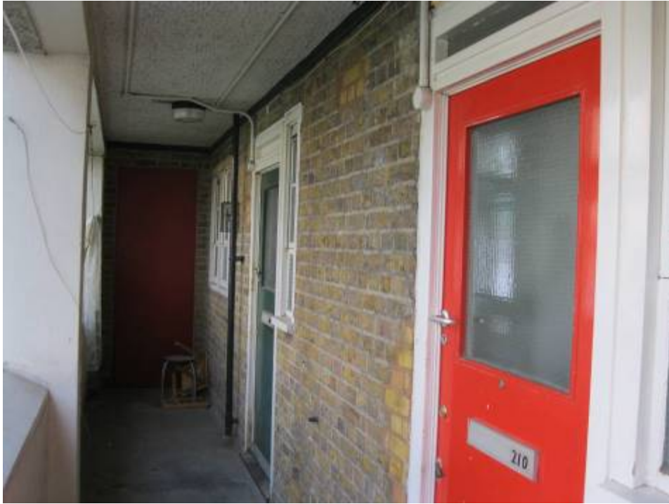
Photograph 27 Typical flat entrance doors
