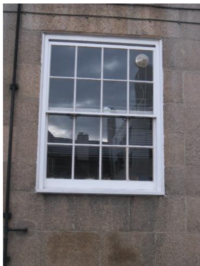
Existing sash window in 1-21 Levita House
