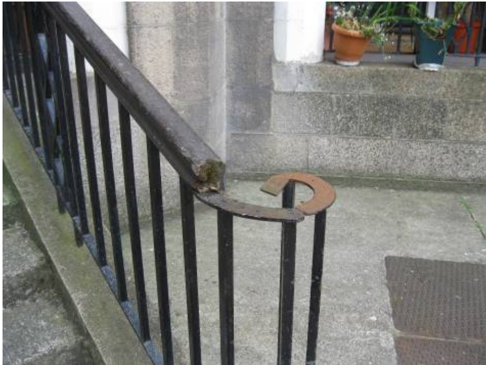
Photograph 39 Entrance steps and handrail 135 - 180
