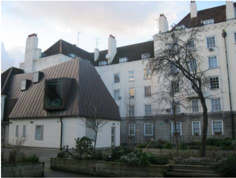
Photograph 5 Rear 204 – 238 showing New Horizon Youth Centre new block
