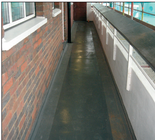
Tordeck™ on-site in London, UK.
