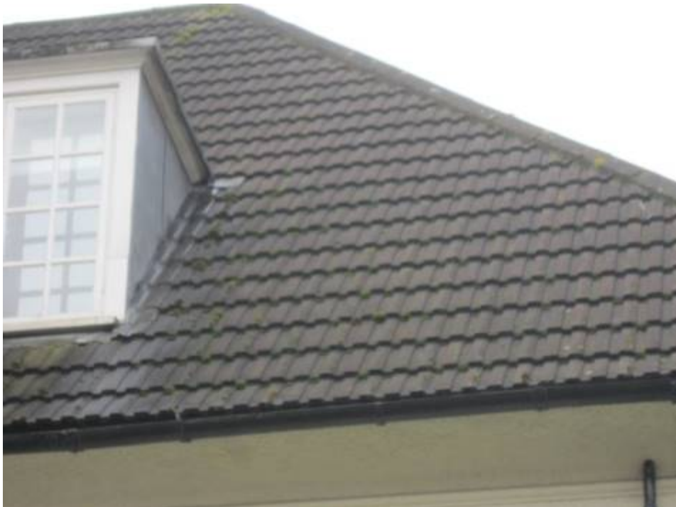
Photograph 2 Recovered roof to 3 storey section of 204 – 238, concrete interlocking tiles
