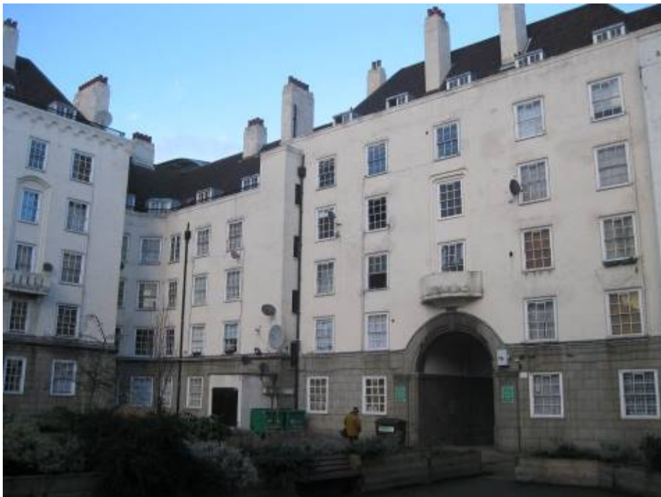
Photograph 6 Rear 183 – 203, courtyard side.
