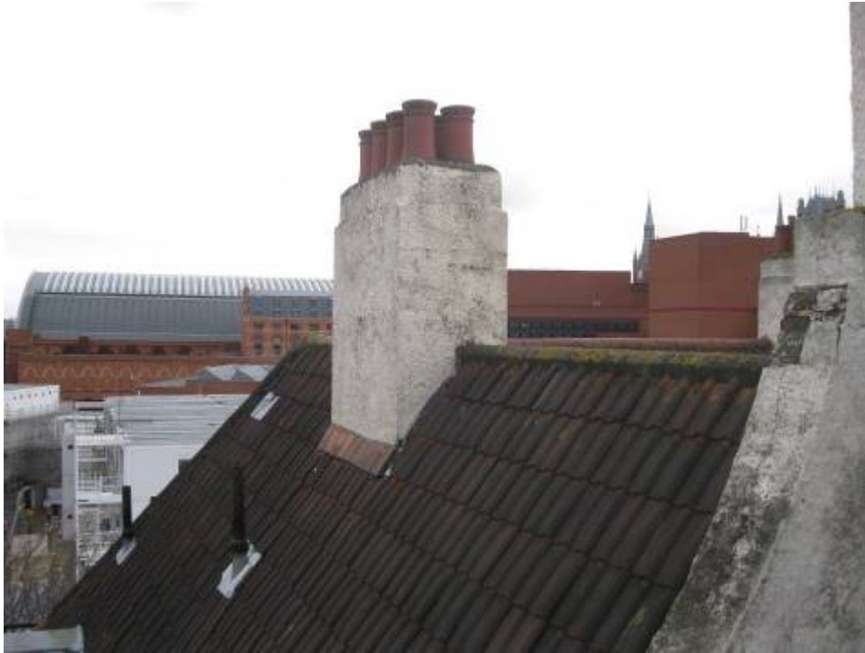
Photograph 9 Pitched tiled roof 204 - 238
