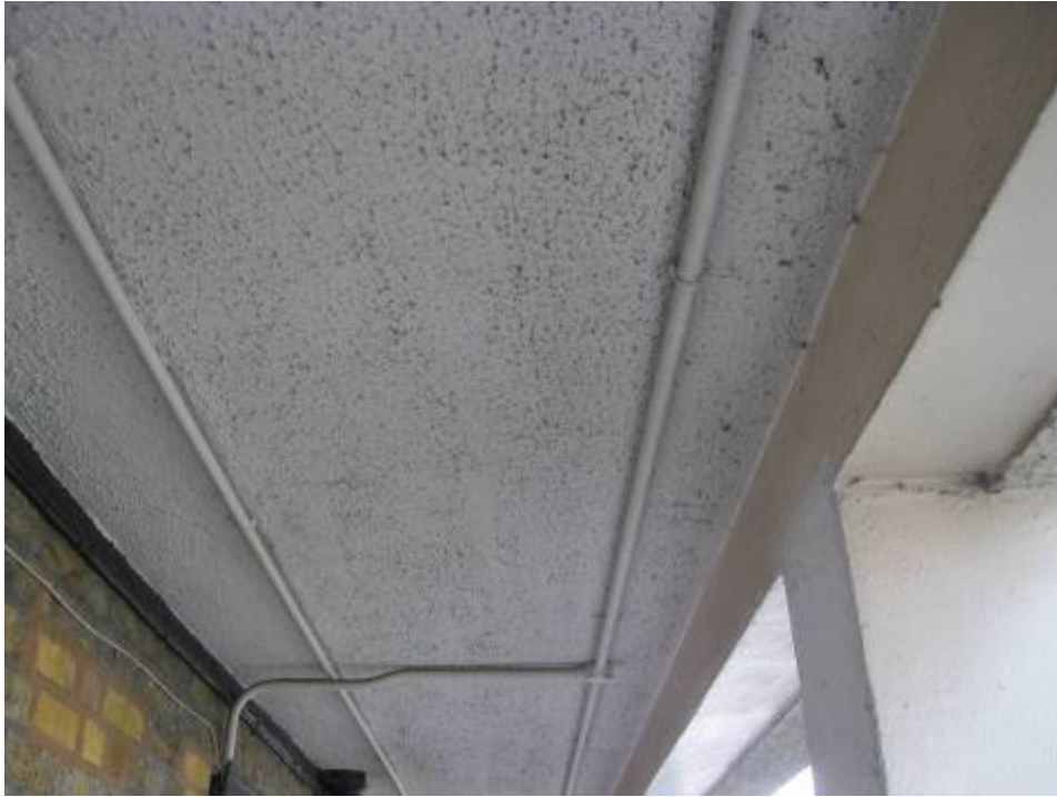
Photograph 23 Access balcony soffit
