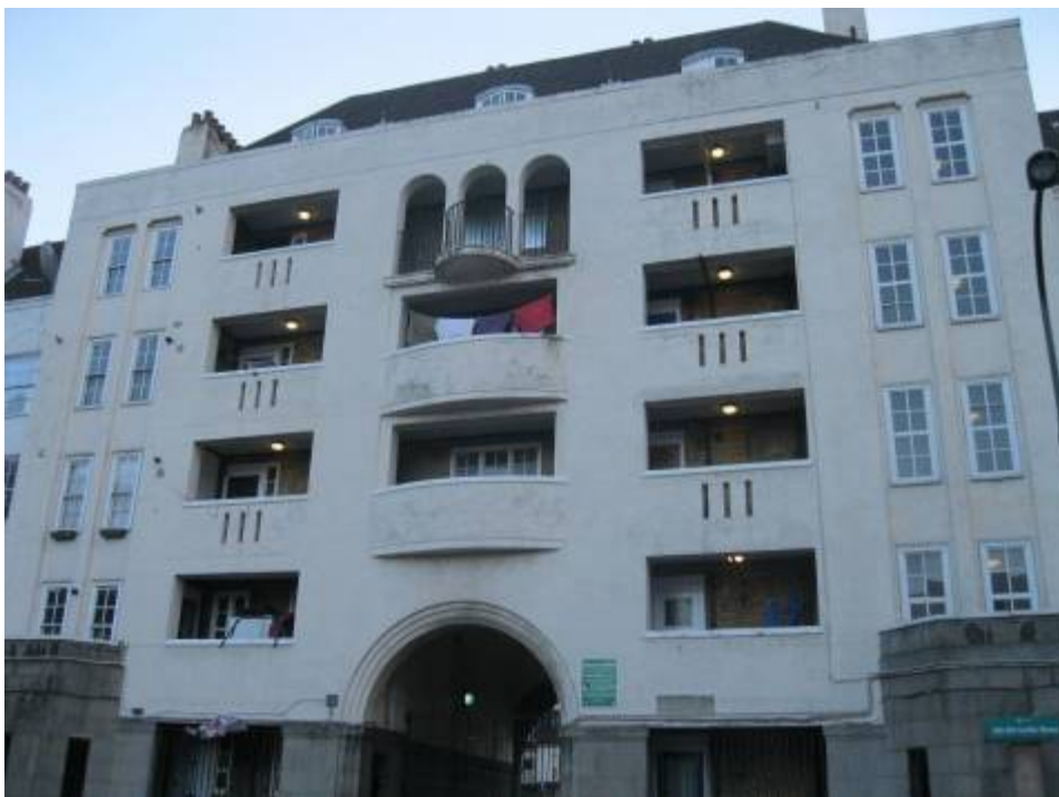
Photograph 8 183 – 203 Ossulston Street Elevation
