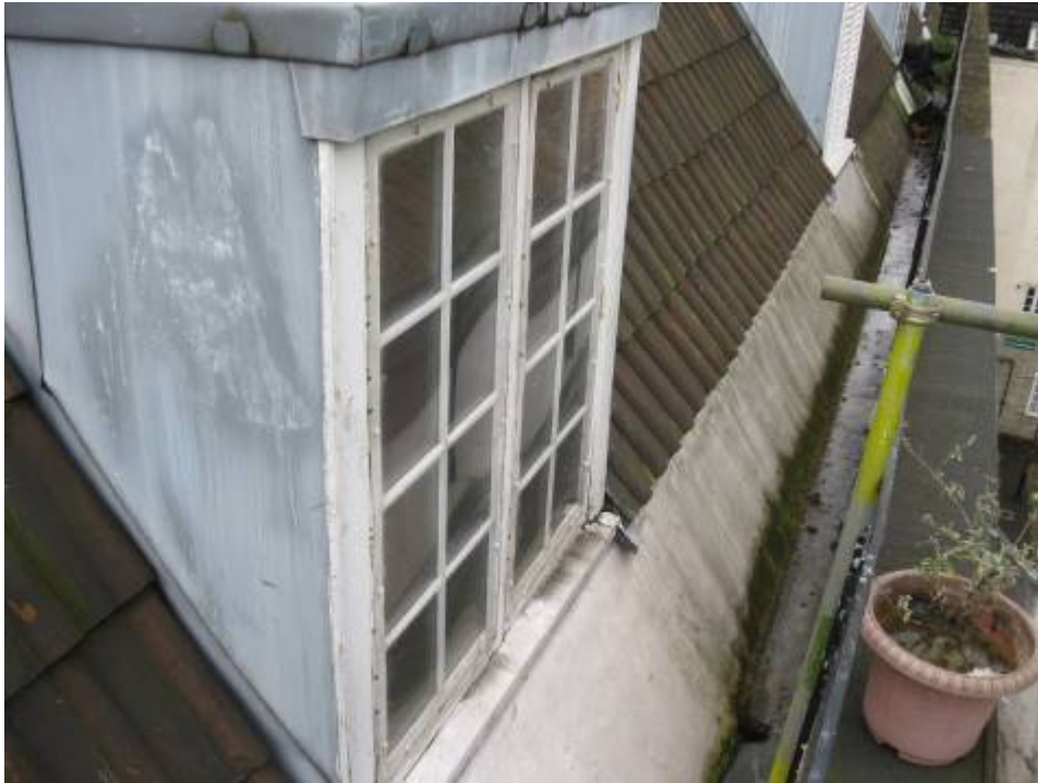
Photograph 19 Dormer window, covered in clear polythene type sheet
