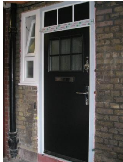
Replacement door fitted in adjacent similar block.
