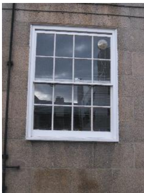
Existing sash window
