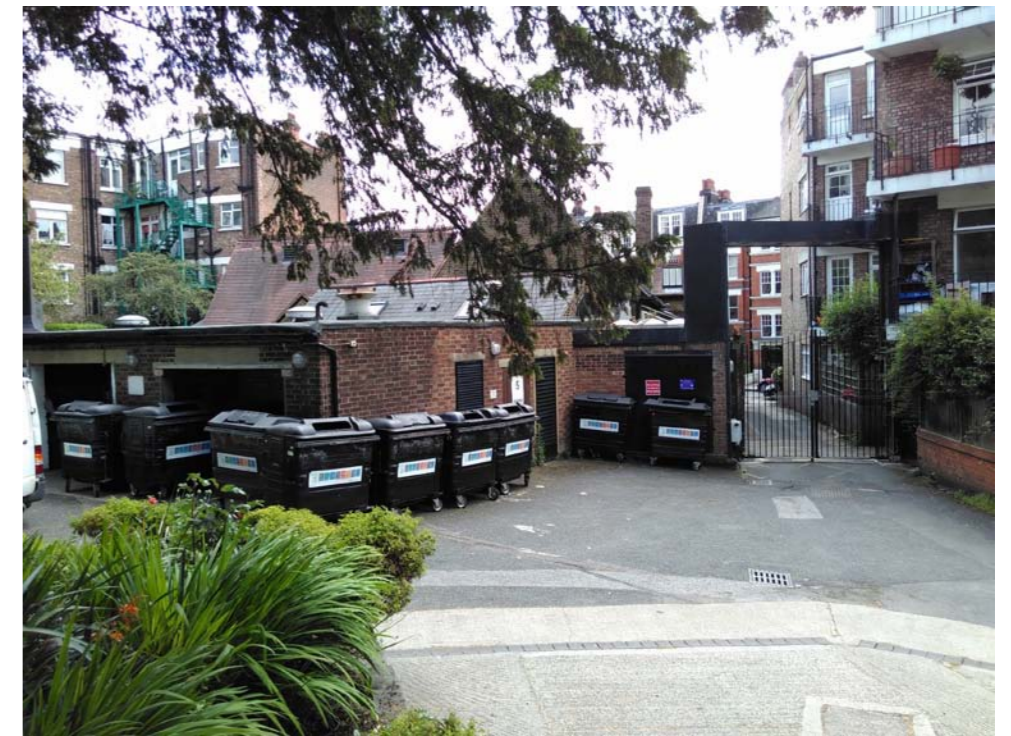
View of boiler house
