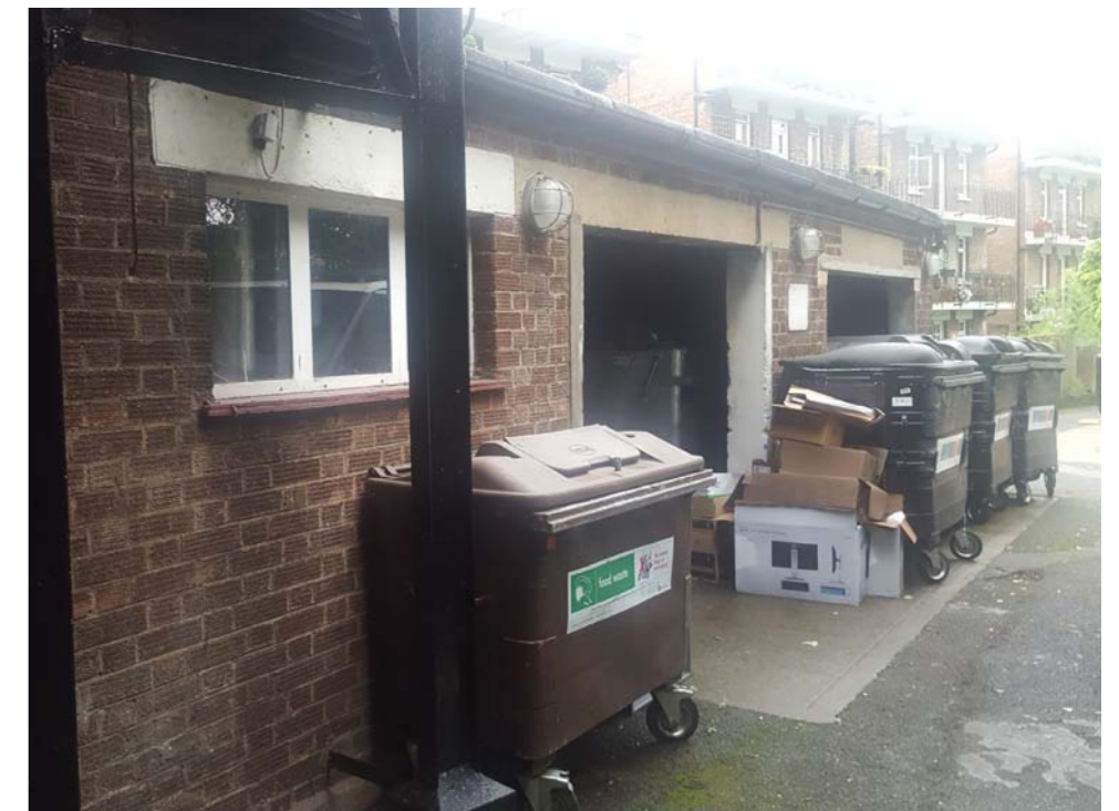
View of North elevation of boiler house
