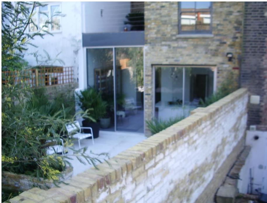
The rear elevation of no. 8, St George's Terrace at ground floor level as existing showing the original garden retained at the same level as the ground floor
