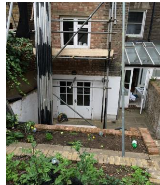
External Joinery and modern conservatory
