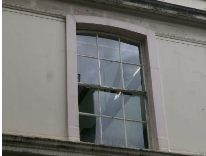
Right Hand Side Elevation – First Floor – flaking decoration and staining to projecting string course.
