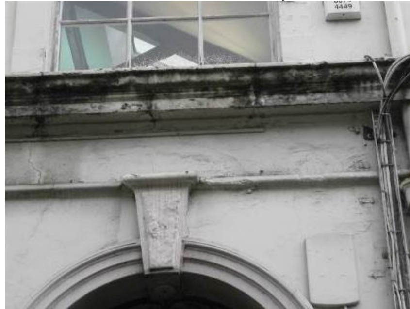
Right Hand Side Elevation - Flaking decorations. Cracking to door heads. Paint-obscured vermiculated render panels.
