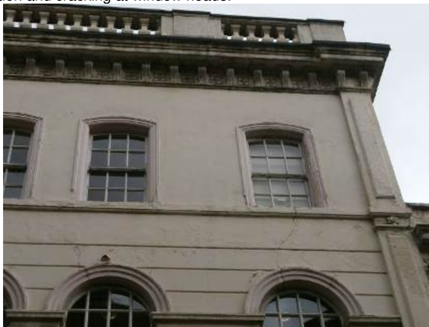
Right Hand Side Elevation – Second & First Floor - flaking decoration and cracking at window heads.
