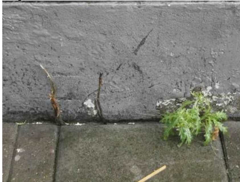
Right Hand Side Elevation - cracking and weed growth to plinth. Flaking decorations.
