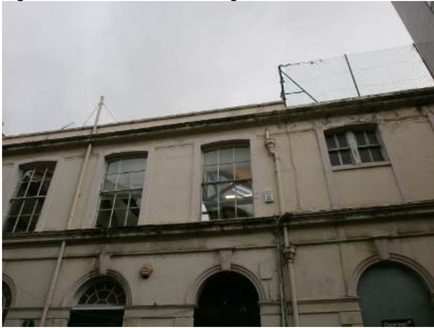
Right Hand Side Elevation – flaking decorations. Cement render at second floor level.
