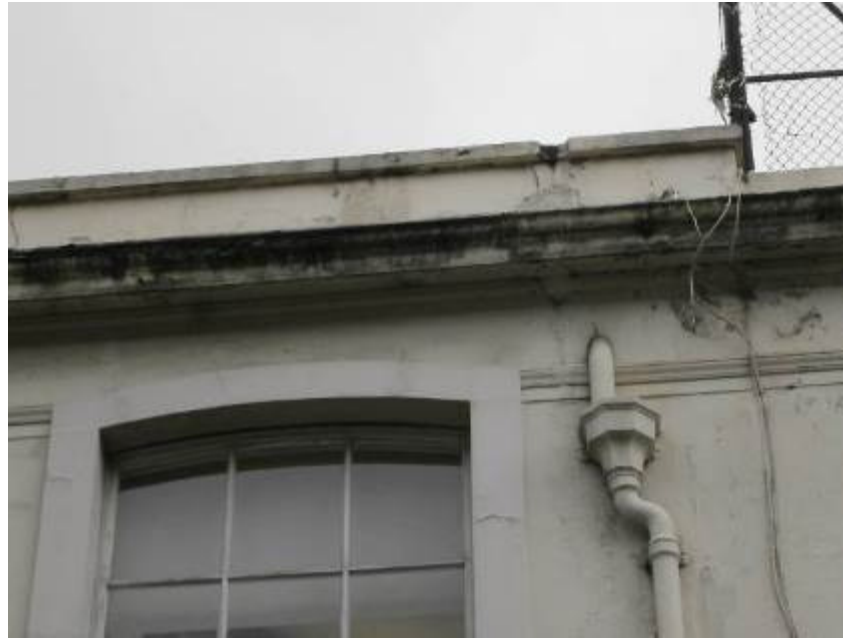
Right Hand Side Elevation – flaking decorations. Cement render at second floor level.
