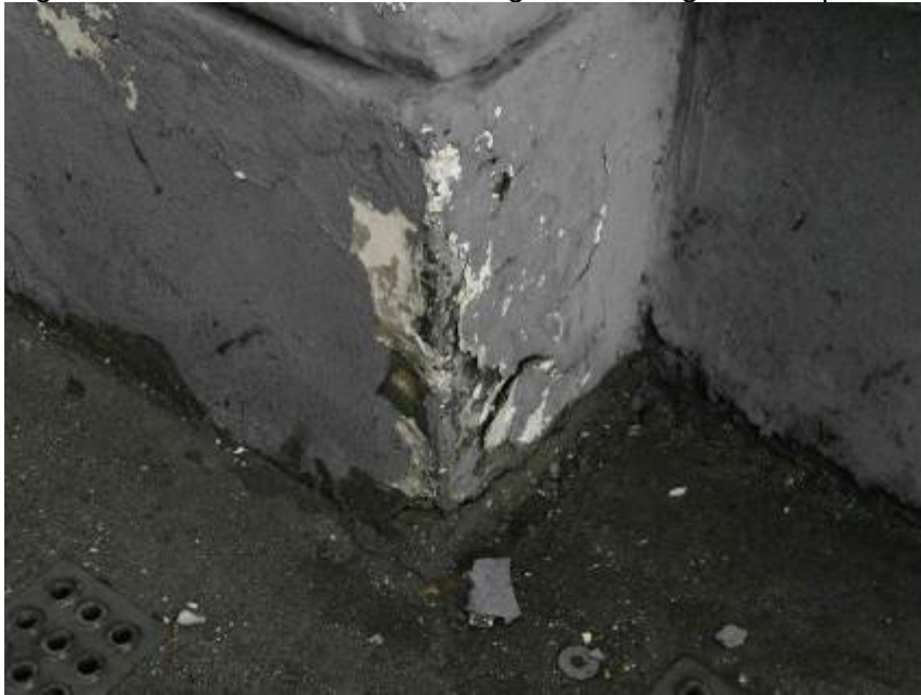
Right Hand Side Elevation - cracking and weed growth to plinth. Flaking decorations.
