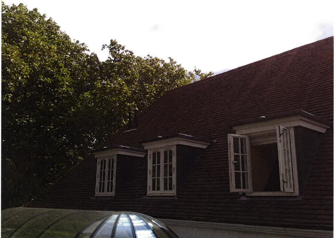
REAR PITCH TO MAIN ROOF - WEST.
