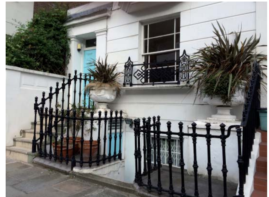
40 Stratford Villas - Main Entrances
