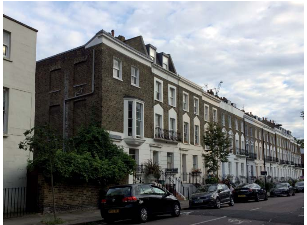
Stratford Villas - Street View
