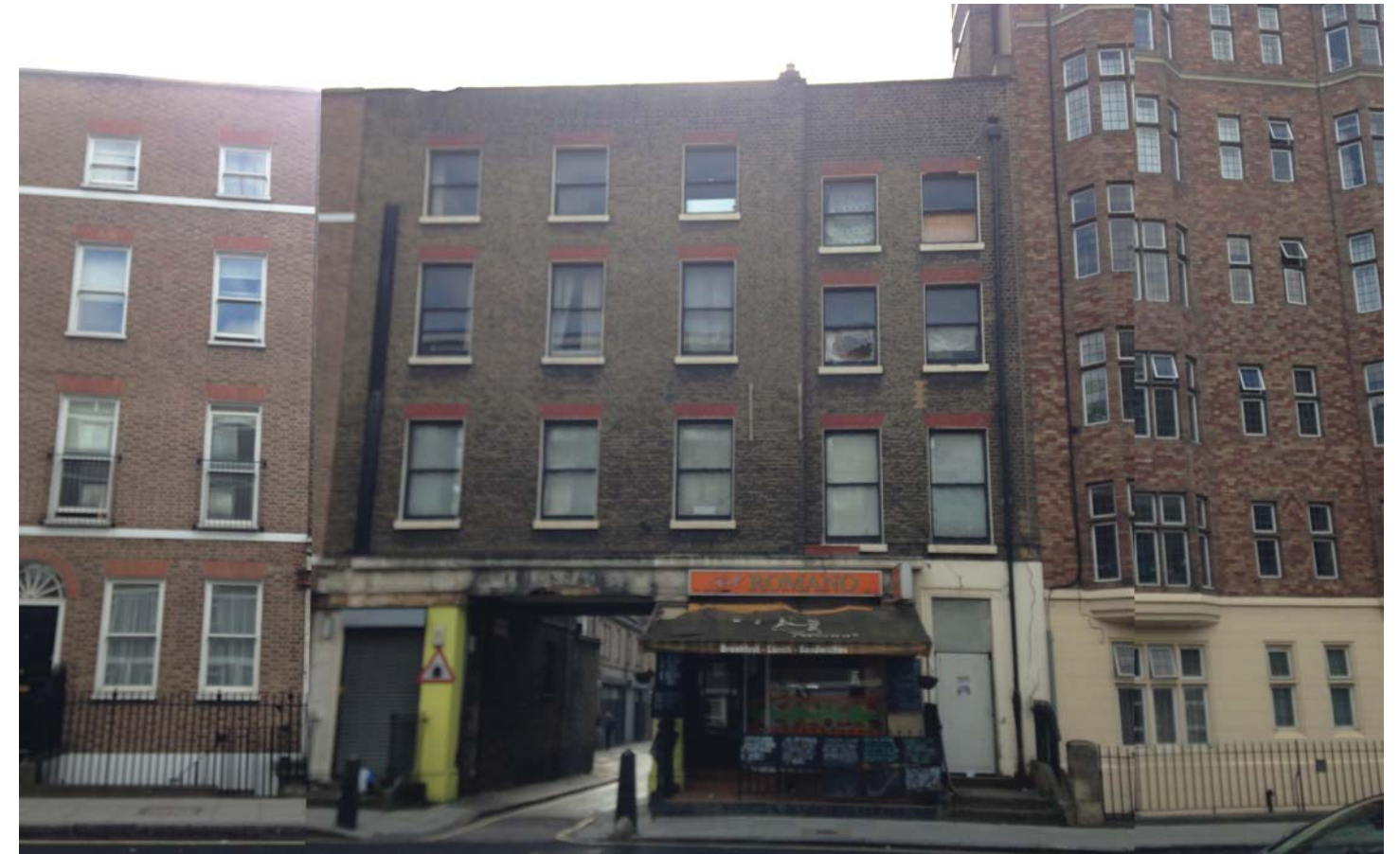
Grenville Street facade
