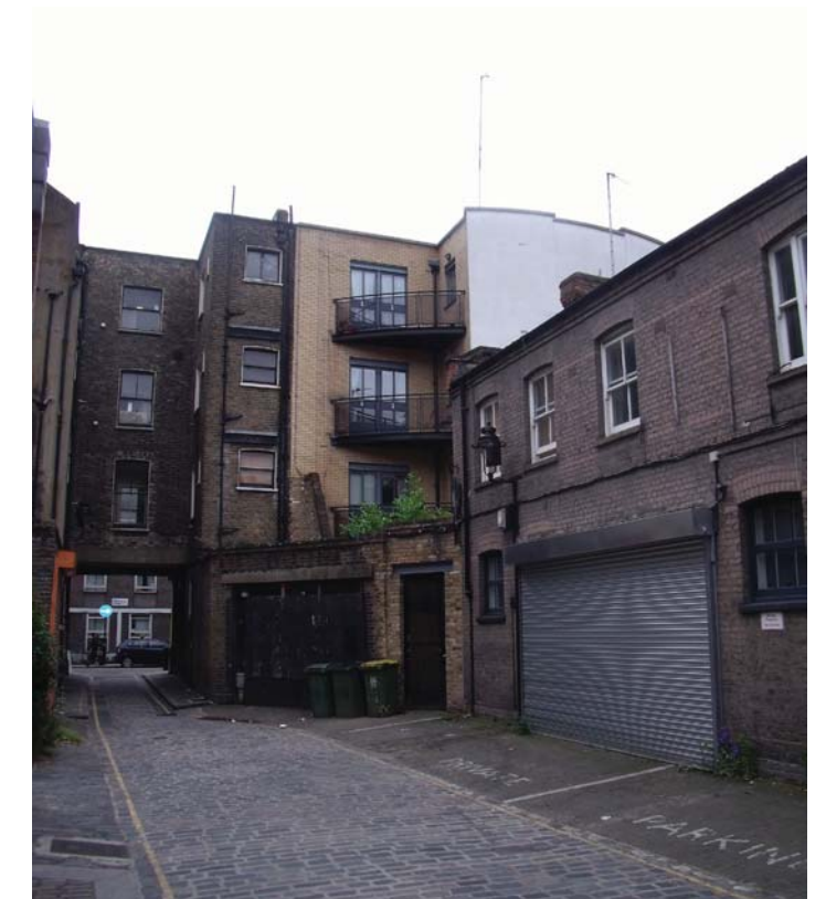
West Facade into Colonnade
