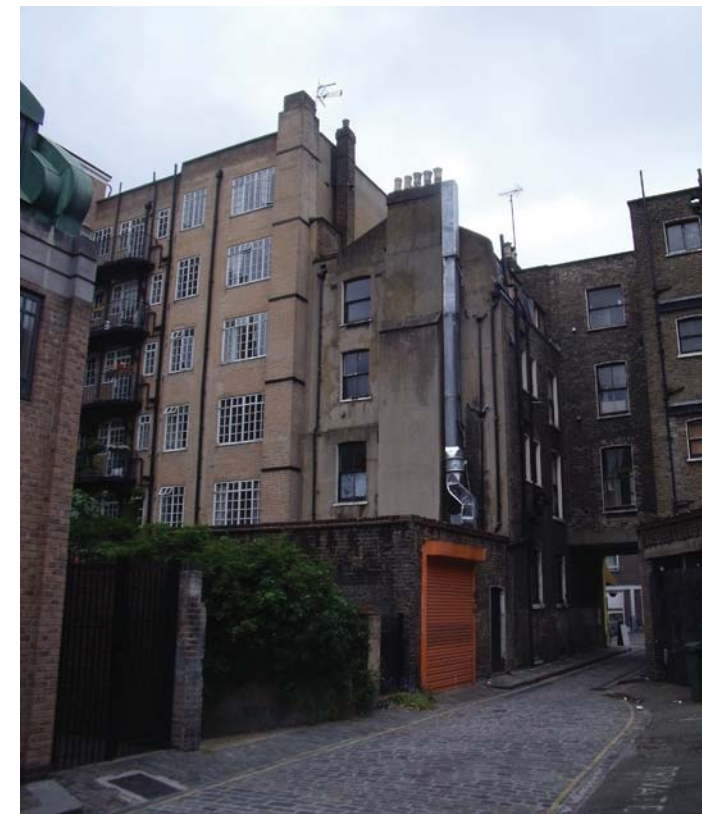
West Facade into Colonnade
