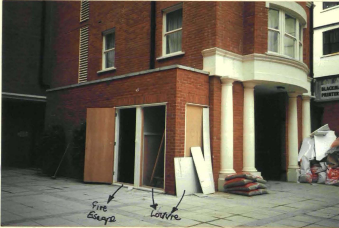
Photo 1 New Stair Enclosure Elevation C. - in drawings 06/8
