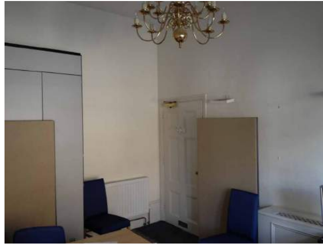
Fig. A34 1st floor - rear office
