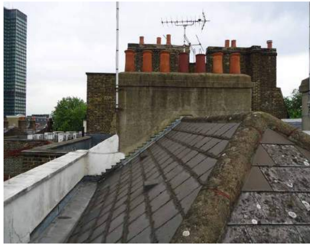
Fig. A48 Main roof
