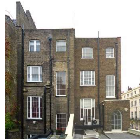
Fig. A4 View of rear elevation
