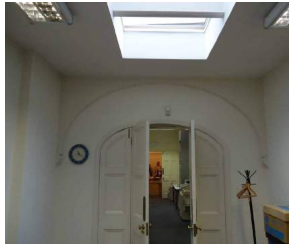
Fig. A22 Ground floor - rear offices
