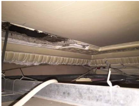
Fig. A36 Original cornice rear room first floor (above modern suspended ceiling)
