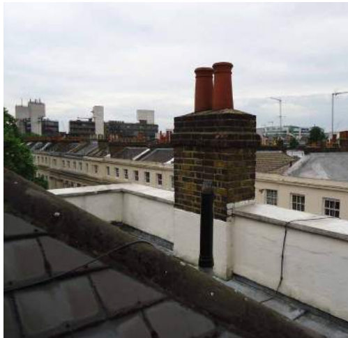
Fig. A50 Main roof
