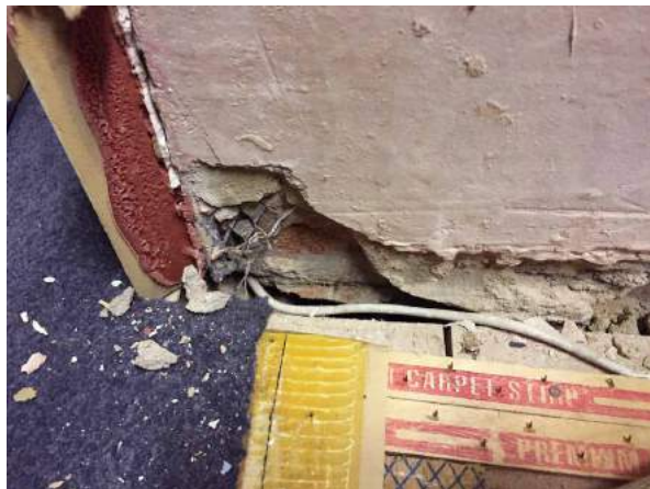
Fig. A27 Recent fletton brickwork and gypsum plaster to rear spine wall
