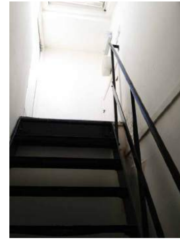
Fig. A44 3rd floor - stairs to roof
