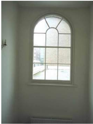
Fig. A29 Ground to 1st floor half landing
