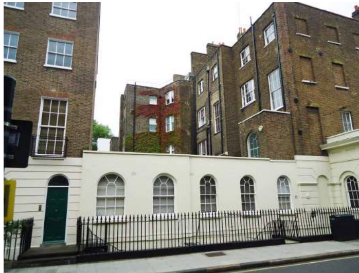
Fig. 8 View east towards 19 to 17 FS from Conway Street
