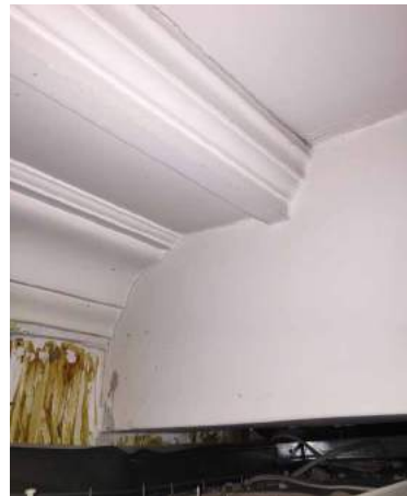
Fig. A37 Original cornice front room ground floor
