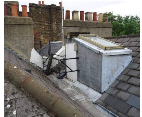
Fig. A49 Main roof
