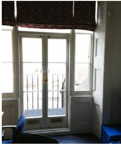
Fig. A33 1st floor - rear office
