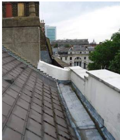
Fig. A51 Main roof
