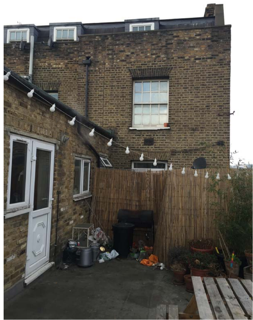
EXISTING TERRACE AND EXTERNAL DOOR
