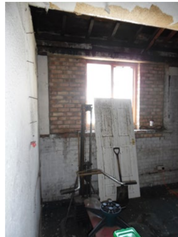
6. Altered window openings
