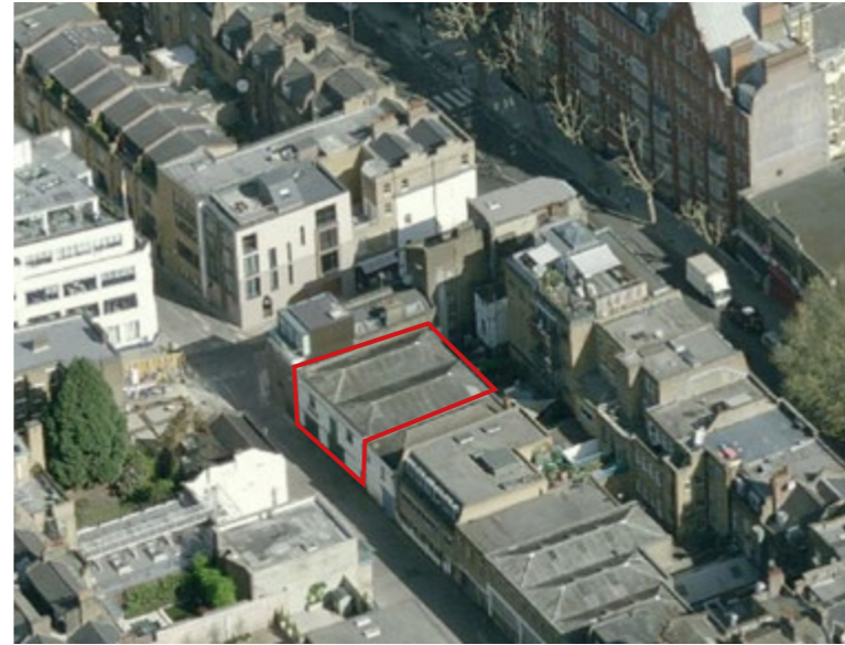
King's Mews and Surroundings Aerial View 02 (Site outlined in red)
