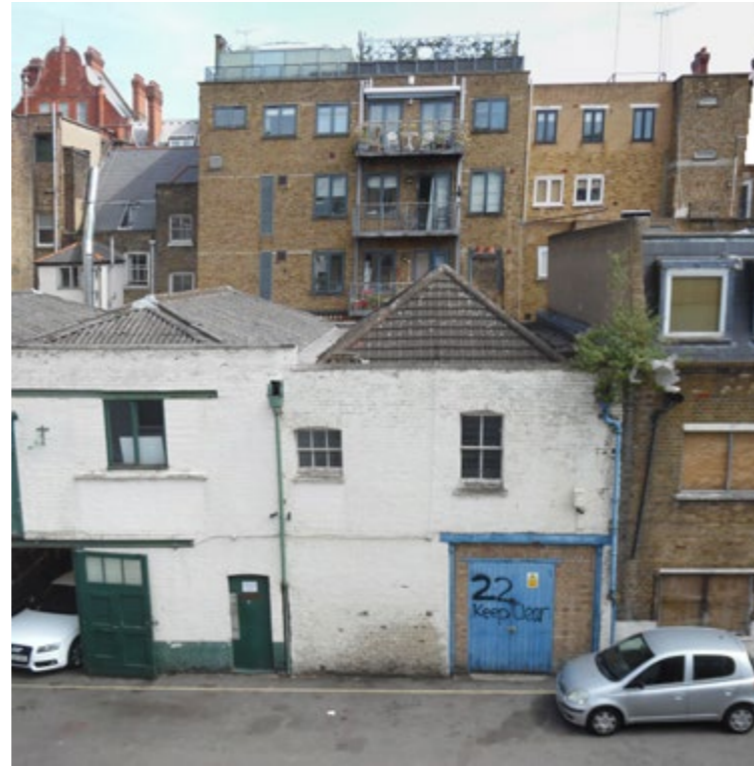
2. Looking North onto the existing site with context
