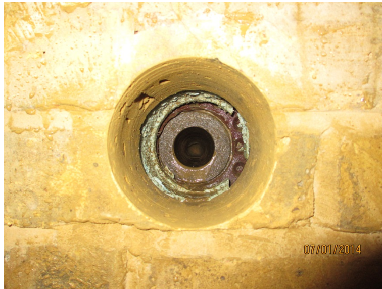
Photo 01 – Typical Core through Existing Wall
