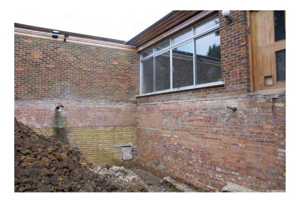
These photographs show the variety of different types of brickwork used in the original construction below the main grade level. They also show the generally very poor quality of the original construction, and the different types of bonding used.
