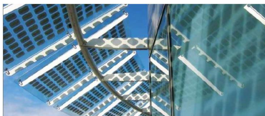
An example of glazing integrated PV is shown in the image above (Romag)
