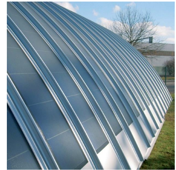
Thin Film Panels installed on the Nation Trust HQ Building in Swindon
