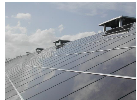
Thin Film Technology Integrated onto an ETFE roof
