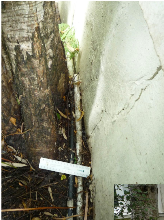
5) Lower trunk showing base touching the wall, vertical crack and broken conduit. September 2015
