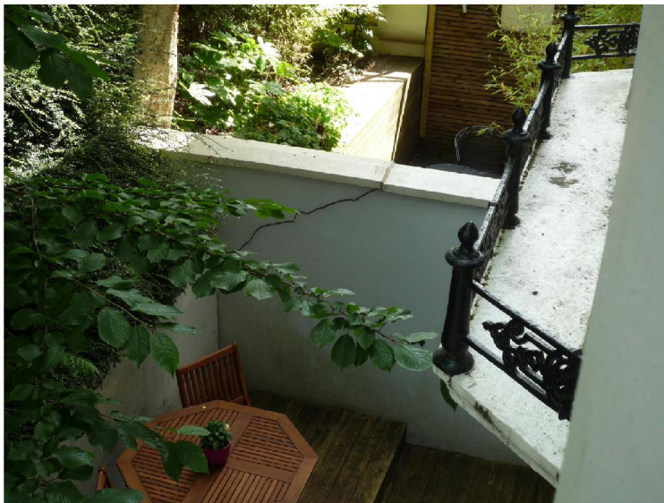
4) Same crack in July 2016, wider although the other side of the wall has been repaired
