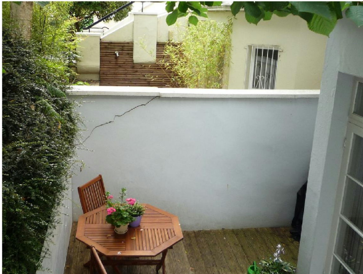
3) View from no.49, September 2015, wider on this side due to the wall being pushed in this direction.
