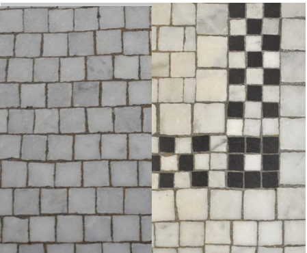
(above) Existing marble flooring and variety of mosaics that appear in small areas around steps
