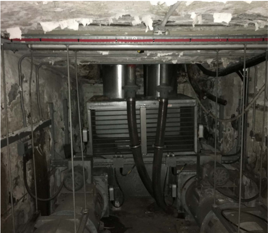
(above) Existing ducted air handling unit within sub-basement tunnels
