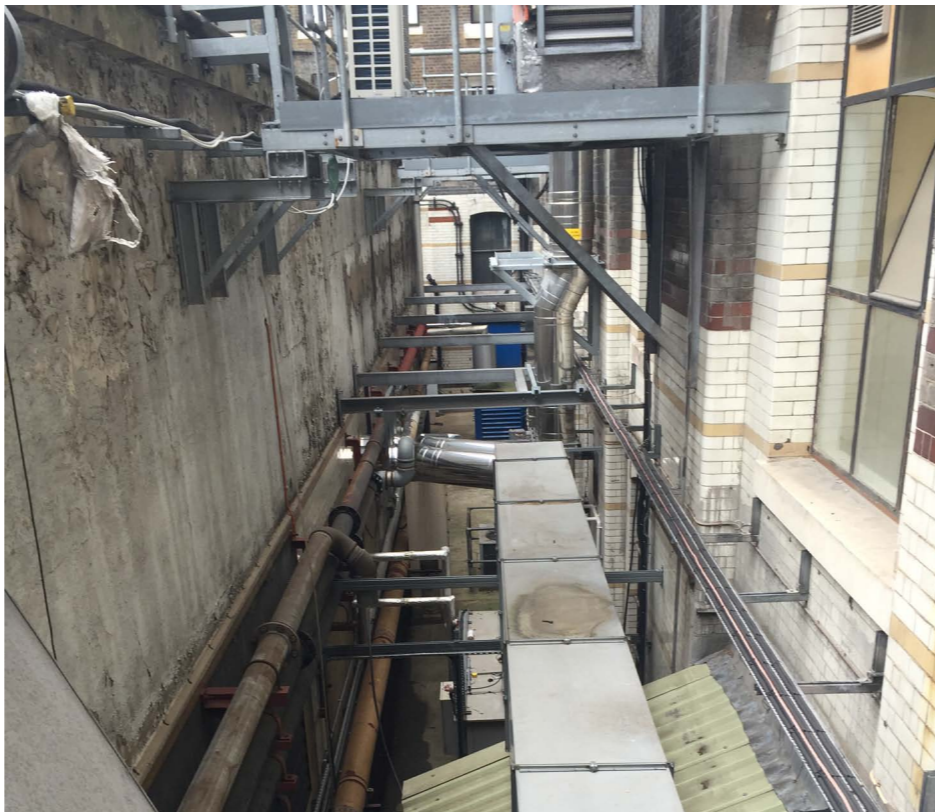
(above) Extensive mechanical plant below existing gallery windows with louvres and vents visible
