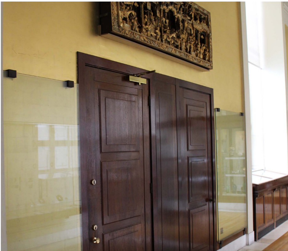
(above) Existing glass protective screens to be retained to vulnerable areas
