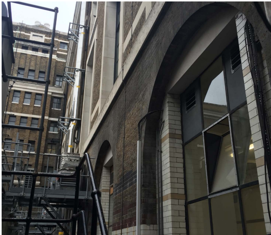
(above) Existing louvres and vents inserted within windows directly below the gallery
