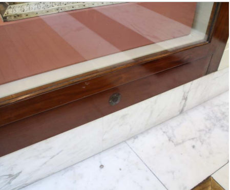
(above) Existing marble skirtings that we proposed to extend across the window openings
