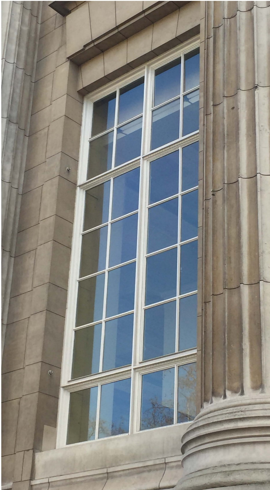
(above) Existing window on north elevation with upper vent visibly unable to close fully
