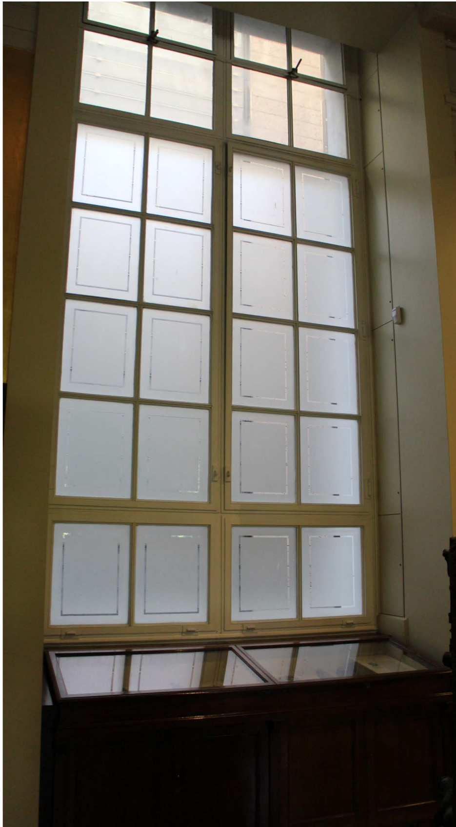
(above) Existing window on south elevation with existing film and teleflex openers to upper vents
