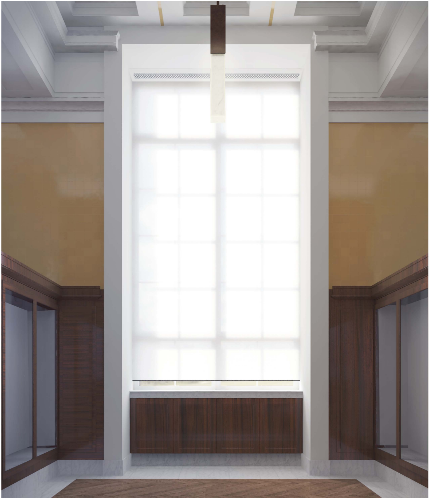
(above) Proposed new bay arrangement with full height blind, new decorative low level boxing, polished white marble cill and high level louvres (south only)
