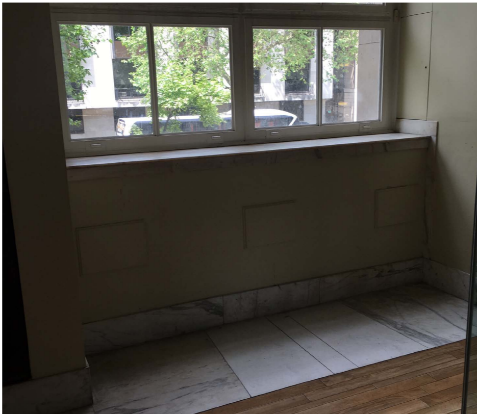
(above) Existing plasterboard infill on the north elevation
