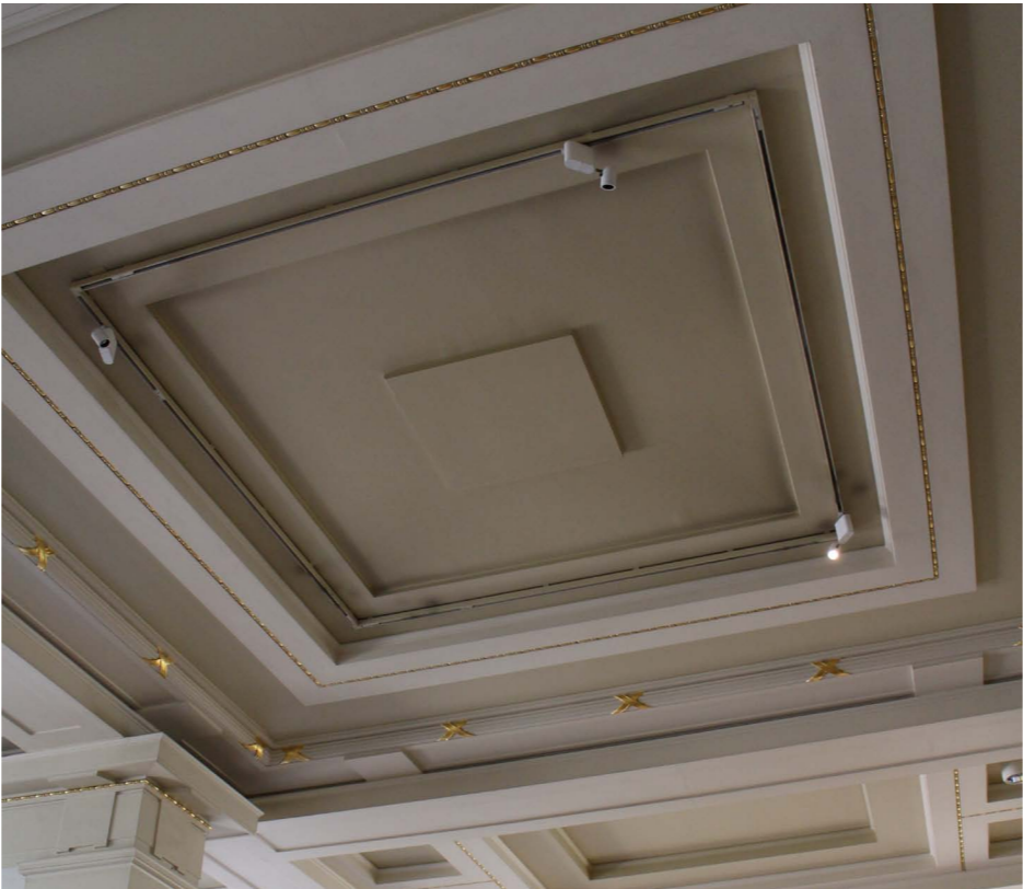
(above, all) Existing plaster ceilings, showing associated mouldings, gilding details and light fittings
