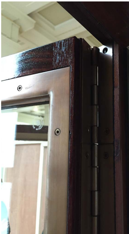
(above) Proposed details for new security locks (top and bottom rails) and bronzed in security frame
