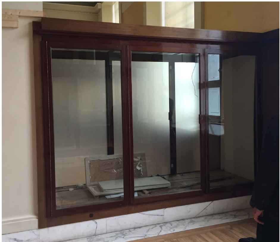
(above) Reinstated but fully openable glazed panels with French polish finish
