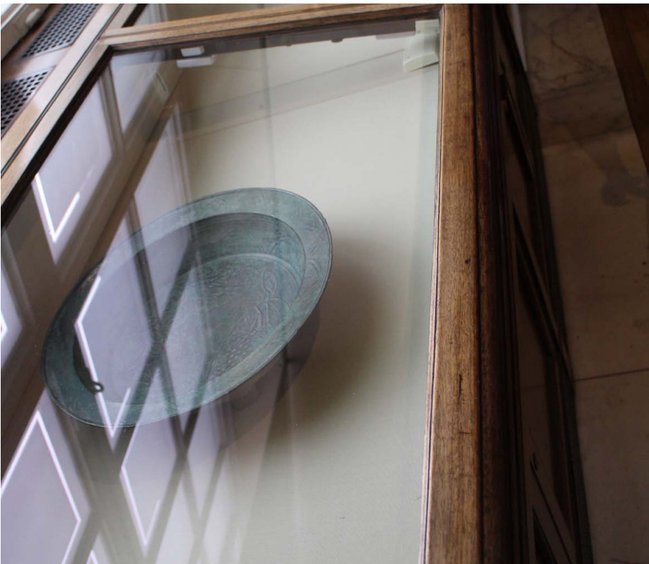
(above) showcase opening mechanism and timber sills with brass ventilation grilles
