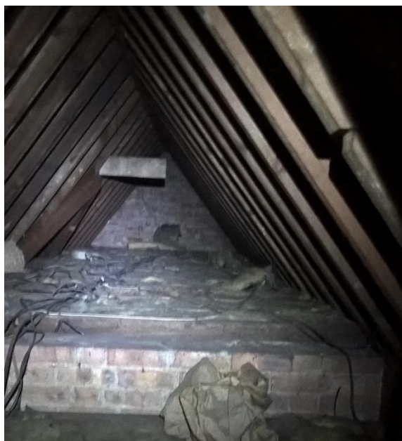
Figure 4.1 typical attic space roof void – wooden boards and intact roofing membranes were observed throughout preventing access into the voids themselves
