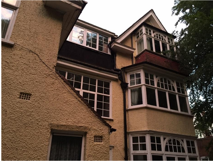
Figure 4.4 28 Redington Road frontage with overhanging eaves
