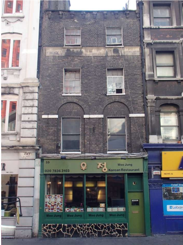
Fig 1: No. 59 St Giles High Street, façade (photo: 2014)
