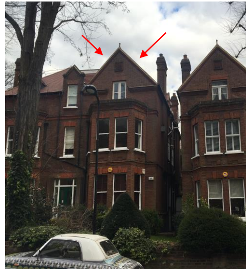
Figure 2. Addition of roof lights
