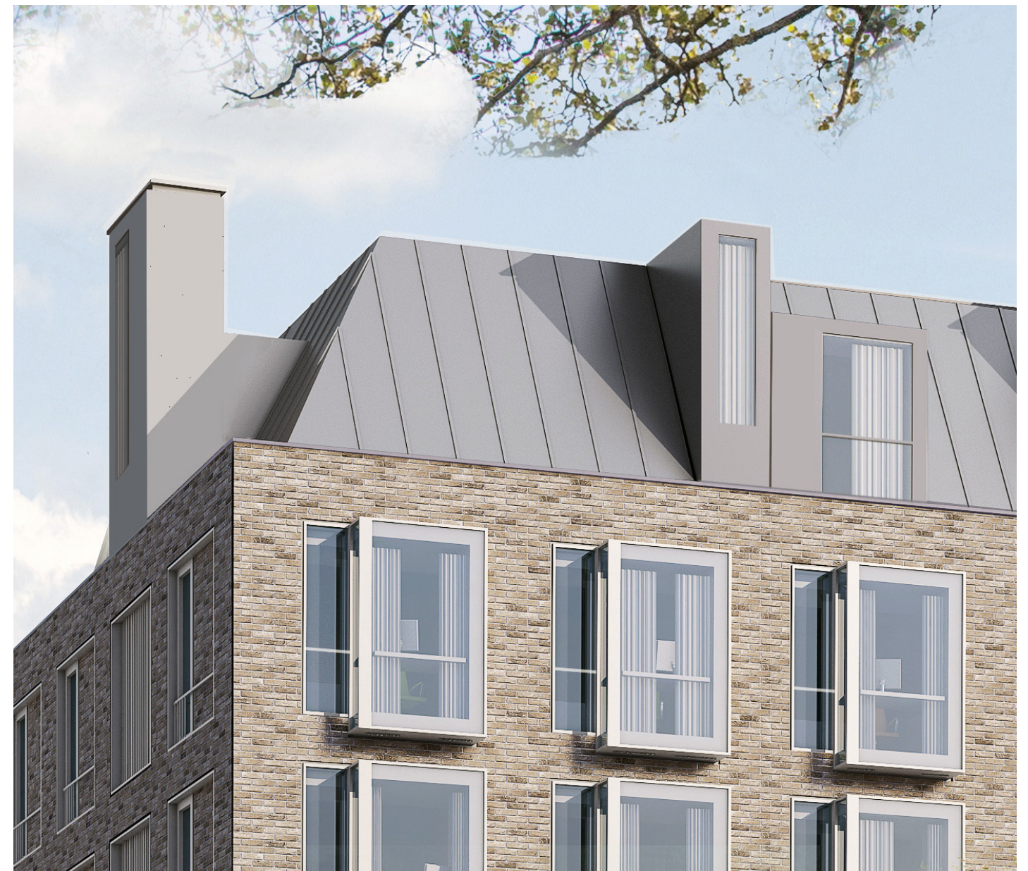
Revised roof proposal showing decreased pitch and raised parapet
