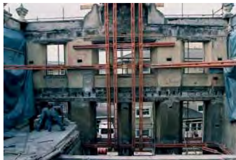
Typical facade retention with walings clamped through windows
