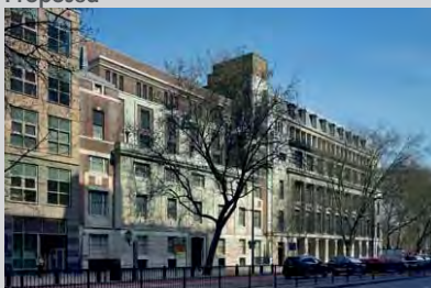
Bentley House (5 additional storeys)
