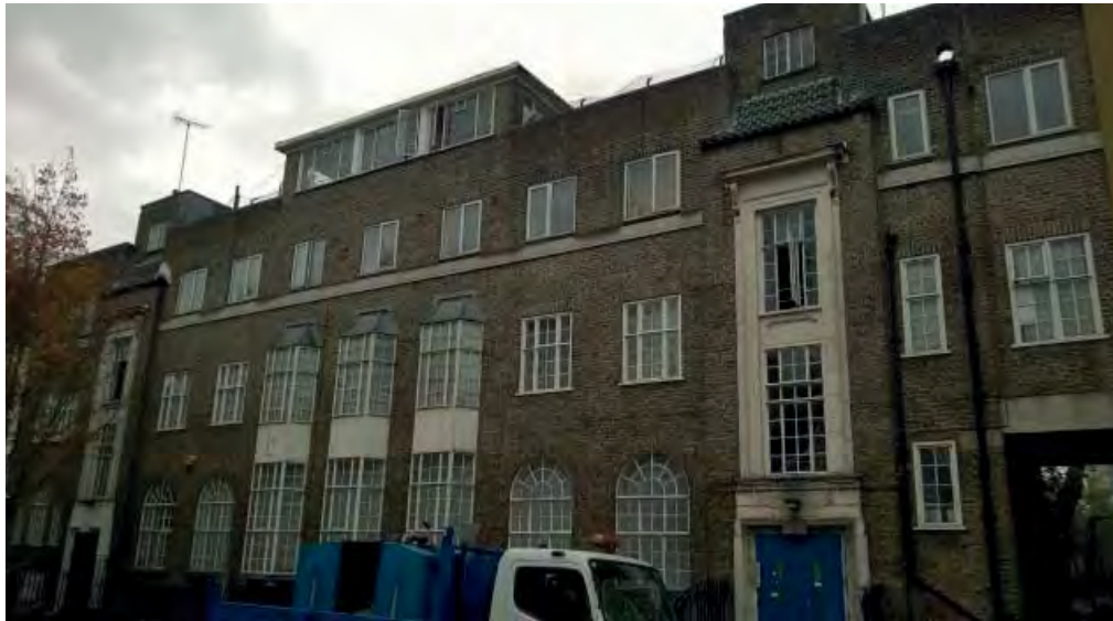
North West elevation of 42 Phoenix Road
