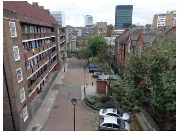
Top floor of existing building, looking south
