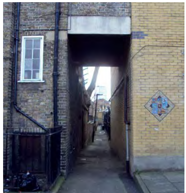
Existing entrance to Clarendon Grove from Phoenix Road
