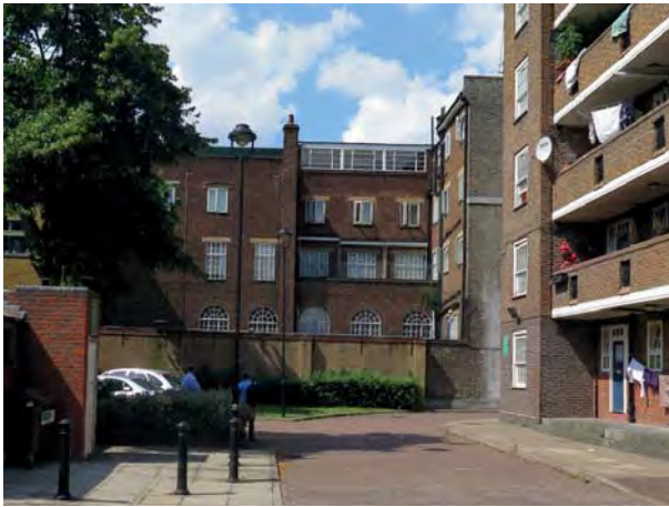
Chalton House Car Park, looking north
