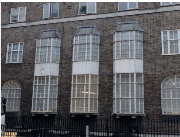
Projecting oriel windows, replaced in the 1960's
