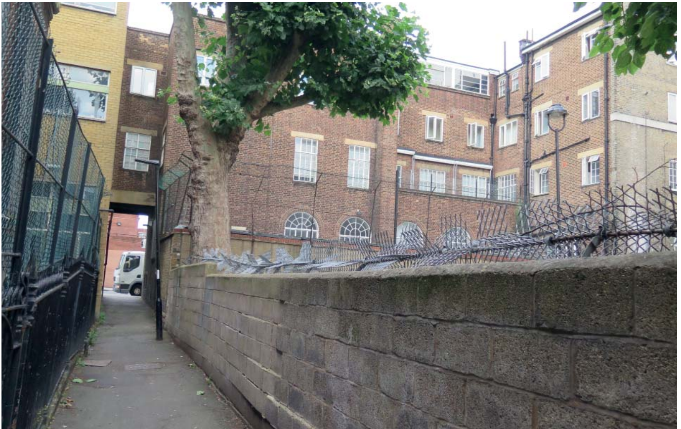
42 Phoenix Road, rear elevation from Clarendon Grove
