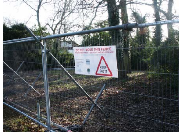
Effective fencing in position
