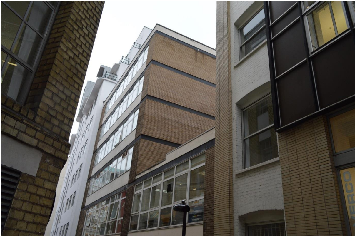
Plate 2 – Onslow Street – Upper levels of rear elevation of building looking south.
