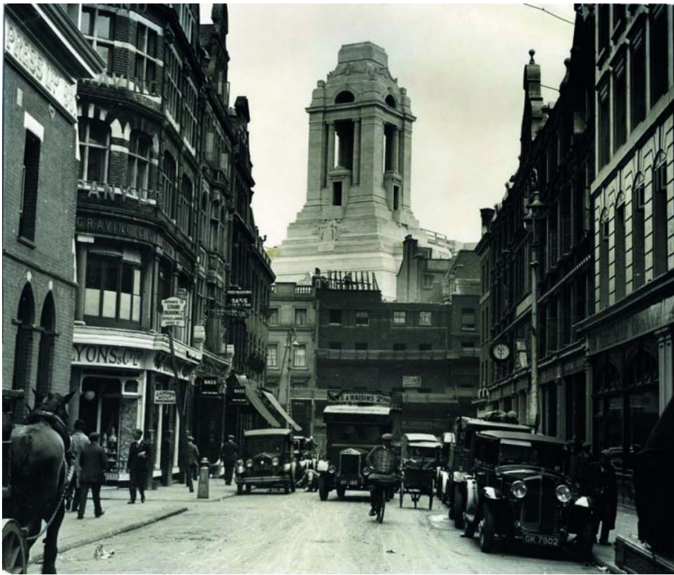
Figure 9: View over partially demolished buildings 1931 (©UGLE)
