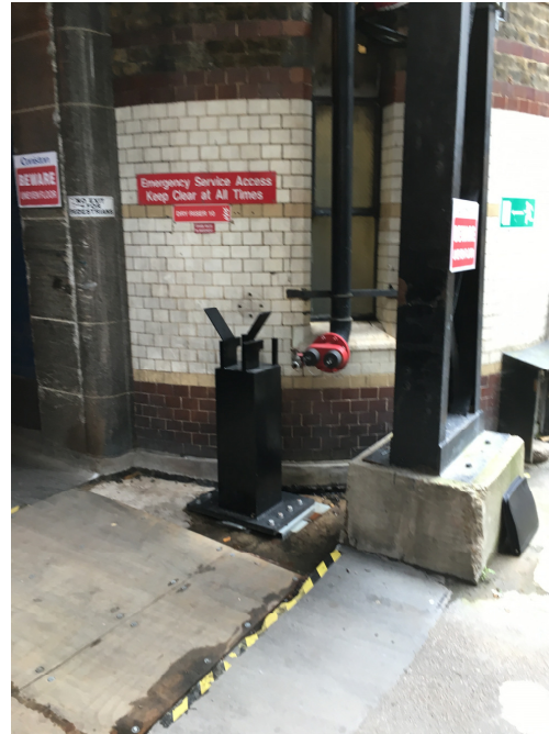
South side showing recent barrier in open position – note barrier rest on right hand side restricting access
