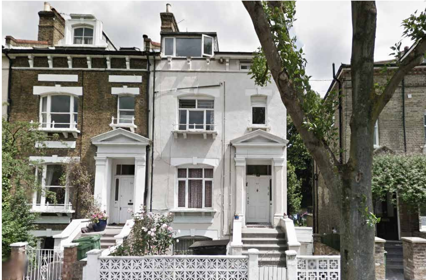
View of the front elevation of the building
