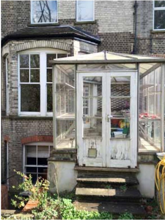
Rear view of no. 40 Arkwright Road, showing existing dilapidated conservatory, rebuilt part of rear wall, and unsympathetic uPVC windows at first floor level
