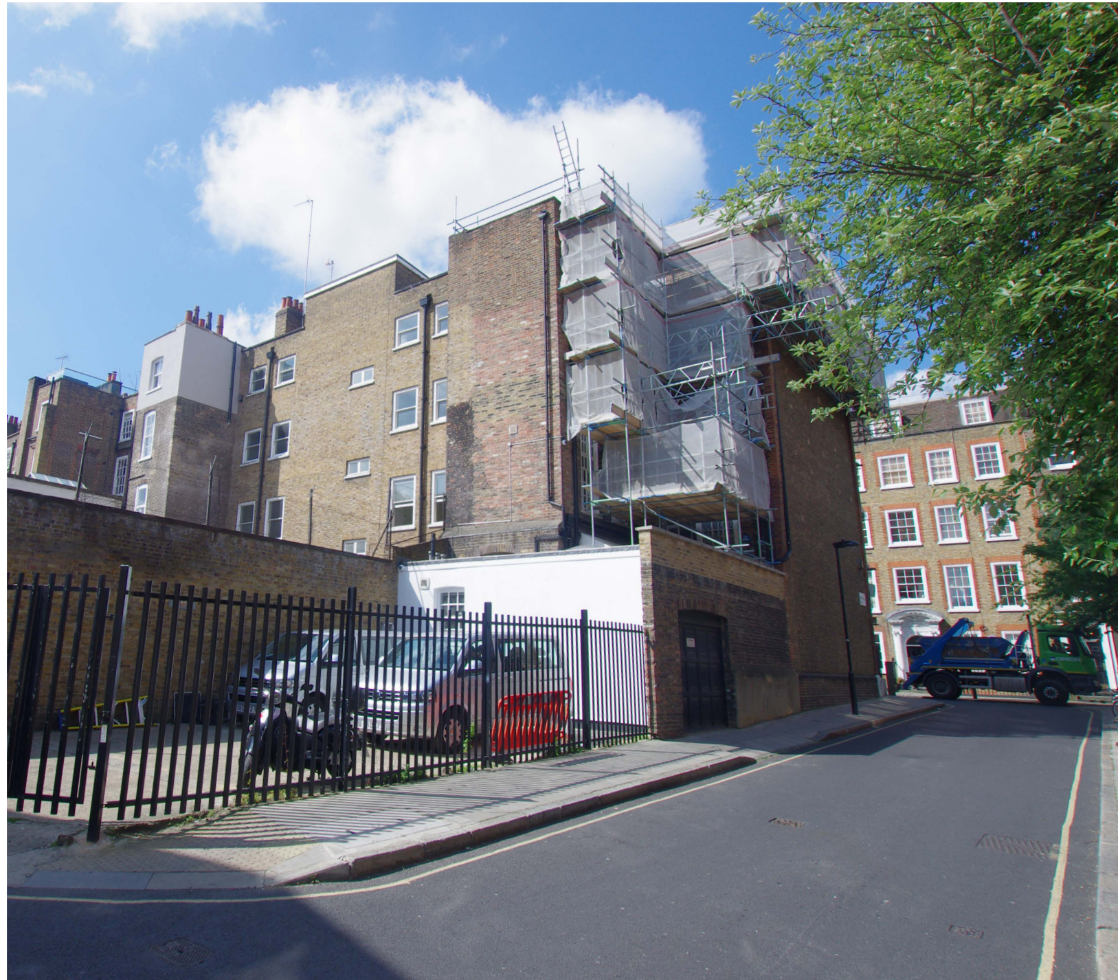
Existing Rear Facade
