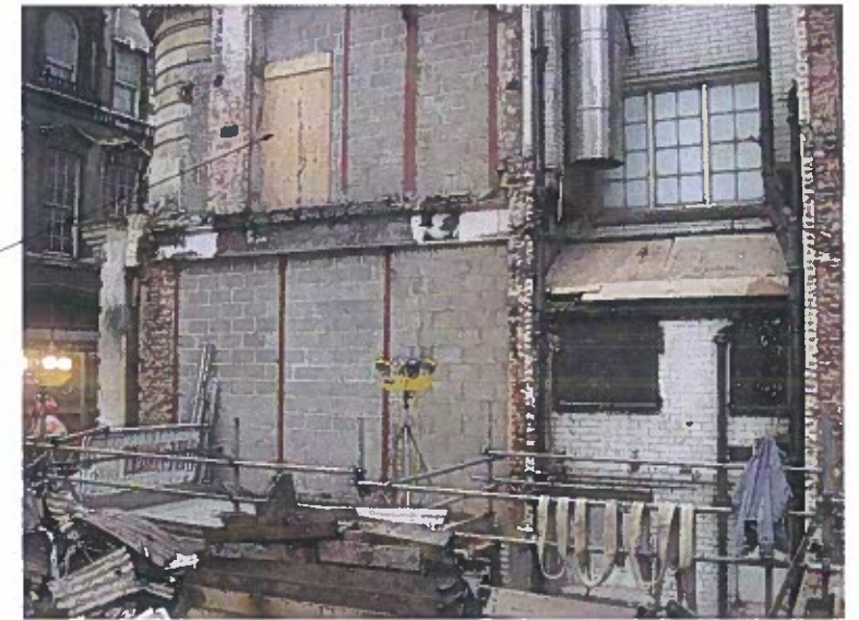
Photograph 1 Indicating existing steelwork and walls to rear of 8 - 10 Southampton Row - South east corner (taken prior to installation of felt and batten waterproofing)
