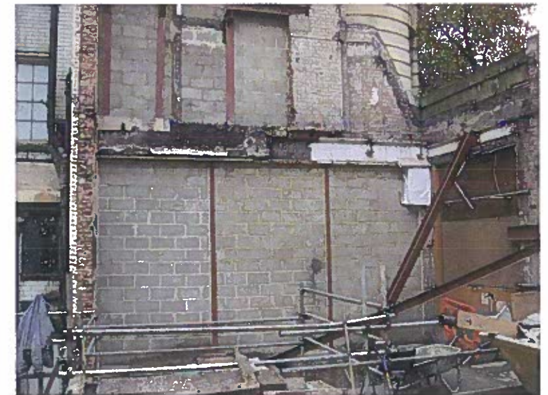
Photograph 2 Indicating existing steelwork and walls to rear of 8 - 10 Southampton Row - North east corner, including props to flank facade (taken prior to installation of felt and batten waterproofing)
