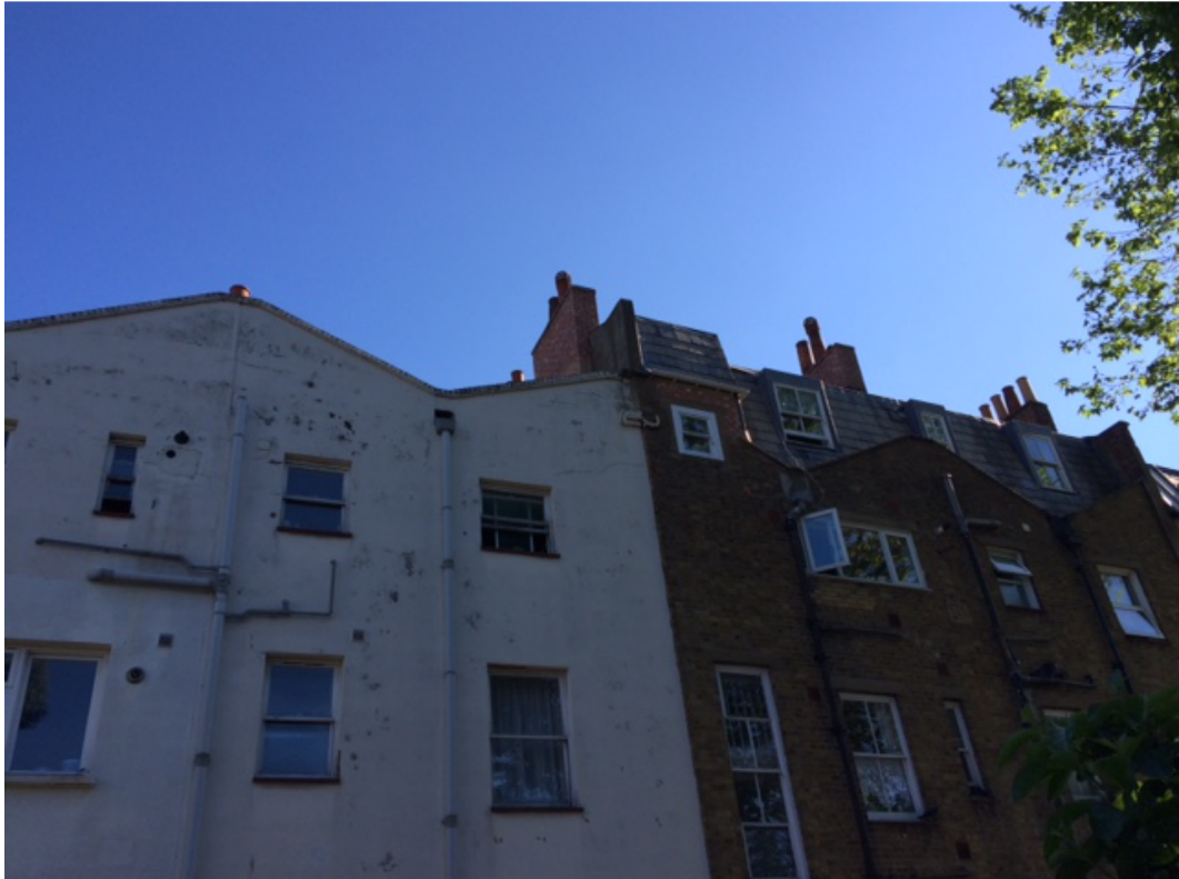
Photo 5: View of rear elevation showing neighbouring property to the south
