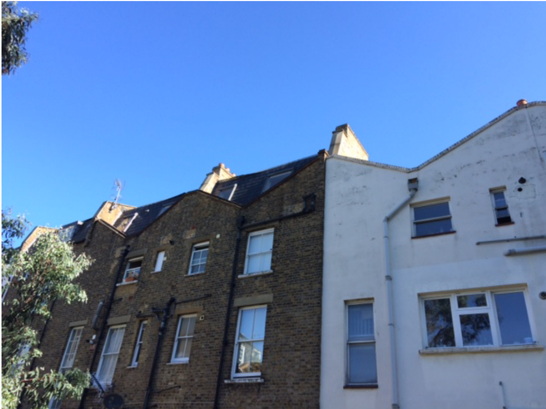
Photo 4: View of rear elevation showing neighbouring property to the north
