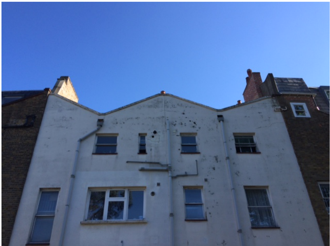
Photo 2: View of Rear Elevation
