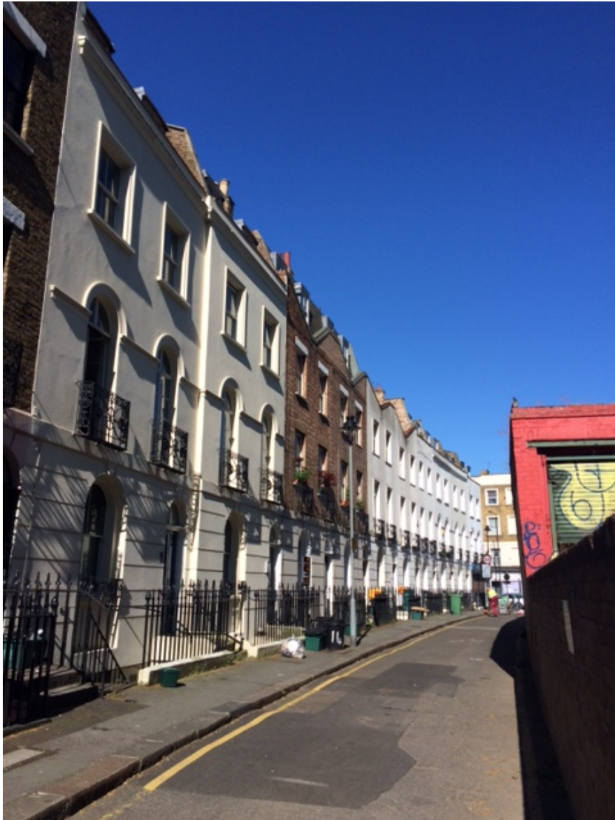
Photo 3: View of existing terrace on St Pancras Way
