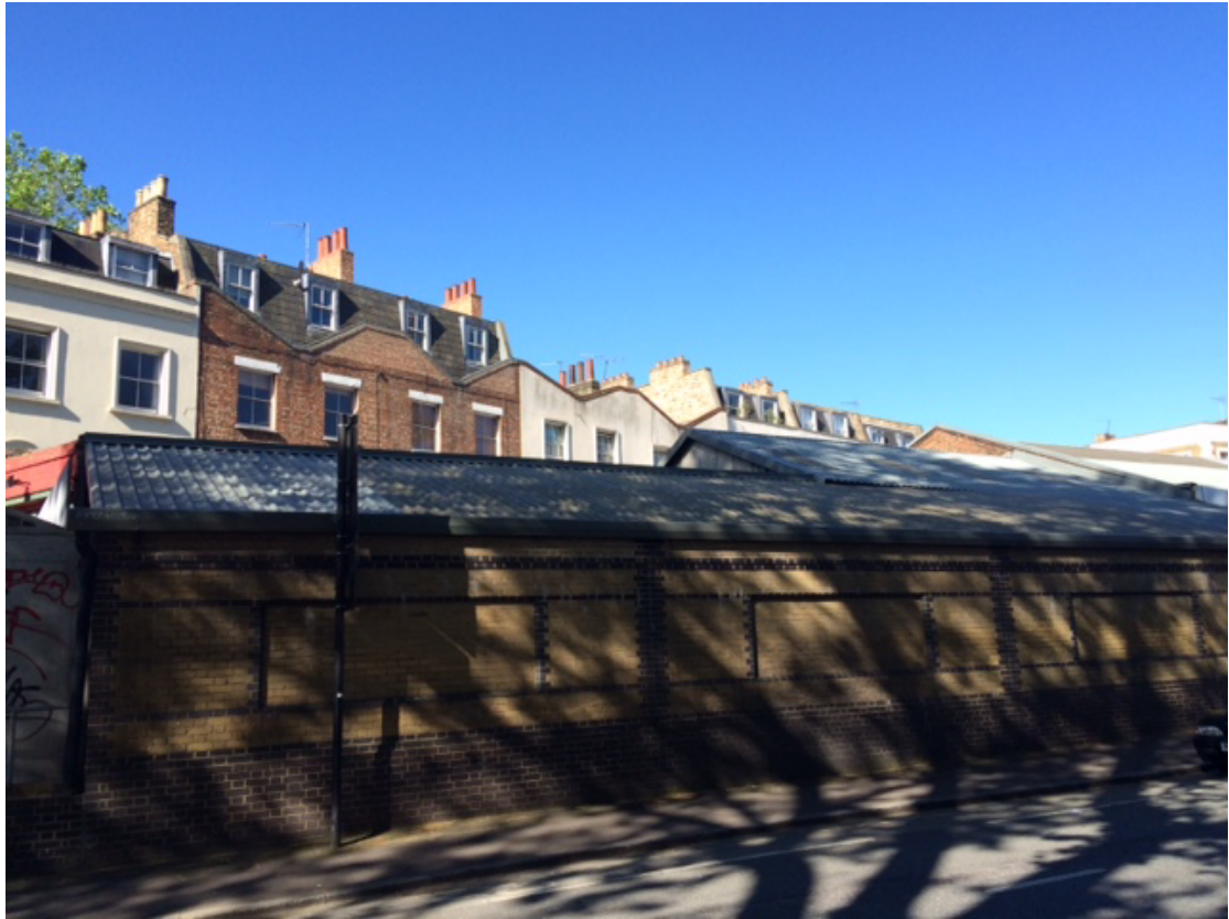
Photo 1: View of site looking west from St Pancras Way
