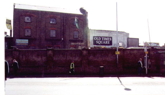
Gin House (Post demolition) Photograph taken 1992
