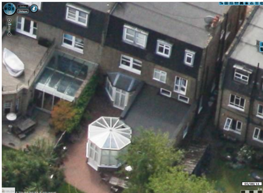
Figure 3 – By standing on the flat roof, the users of the terrace have views back into other floors of the host property and neighbouring windows also.
