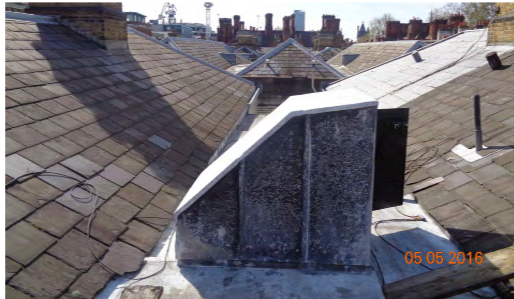
Existing Loft Access Hatch Photo Facing South
