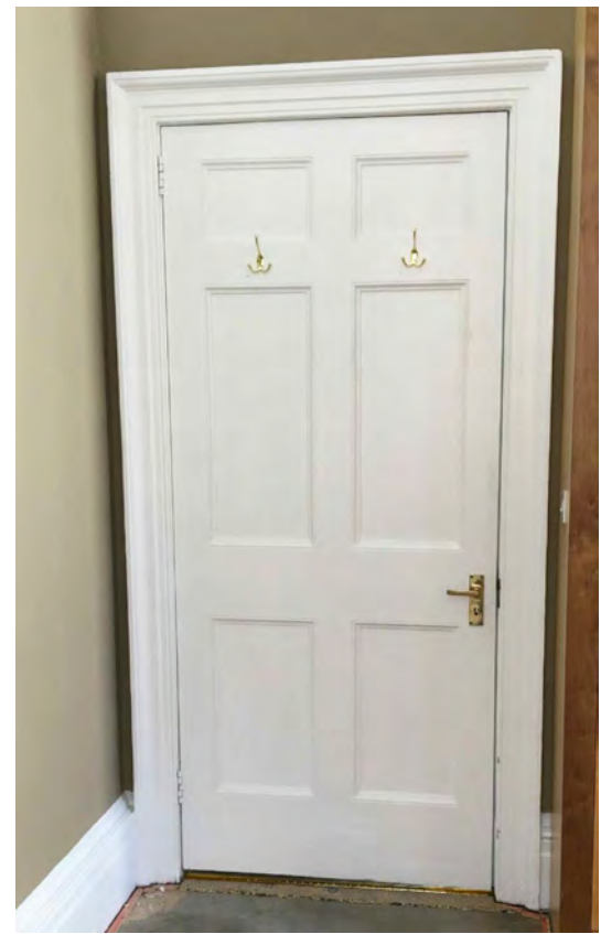
Photo of Internal Door
