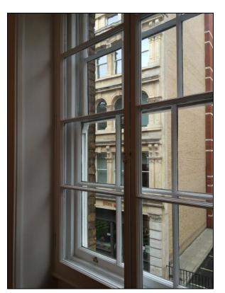
Figure 6 Existing secondary glazing
