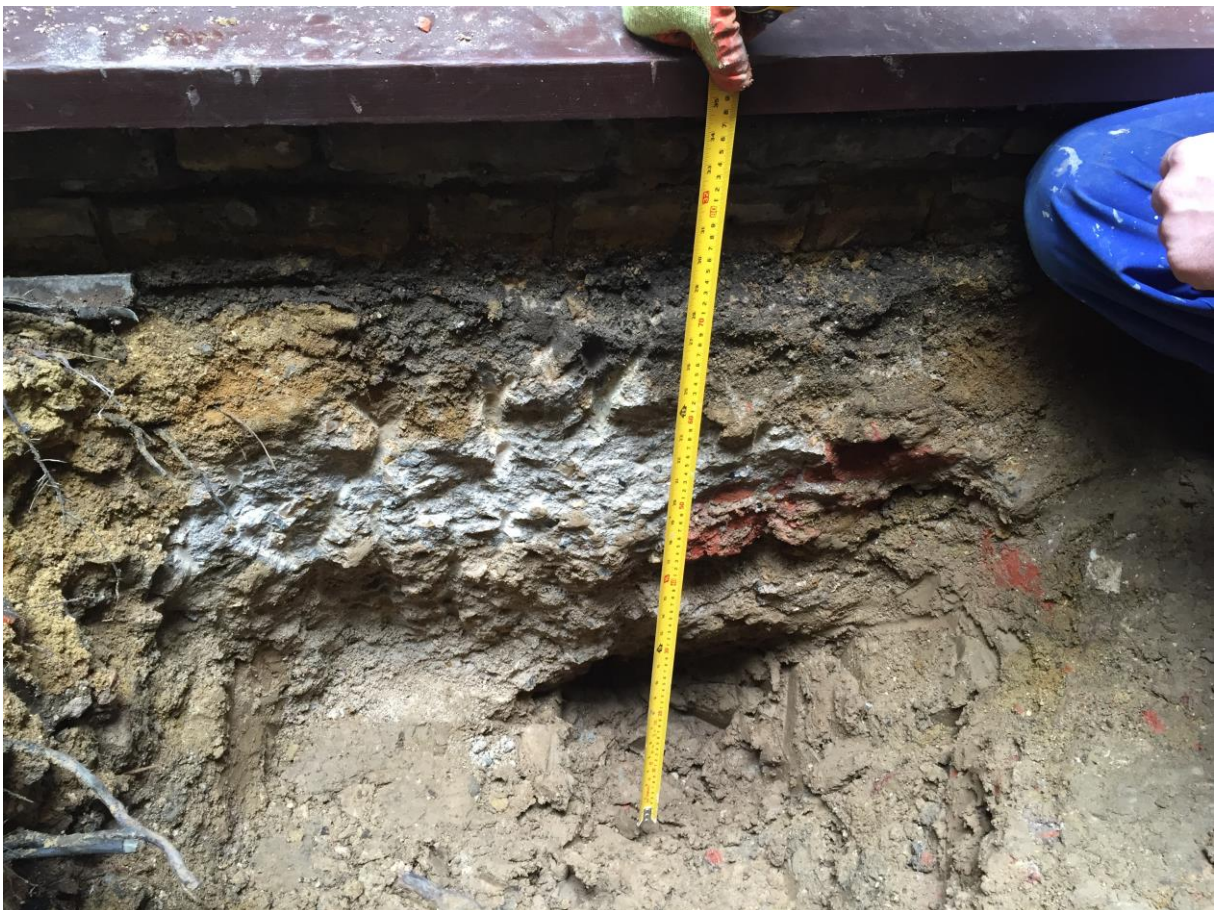
Trial Hole Investigations.
