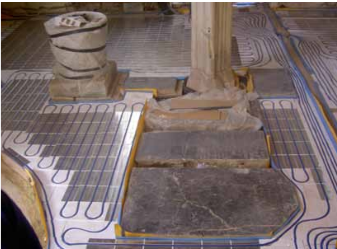
05 The addition of an insulation layer is an essential part of an under-floor heating system © Jupiter Heating Systems
