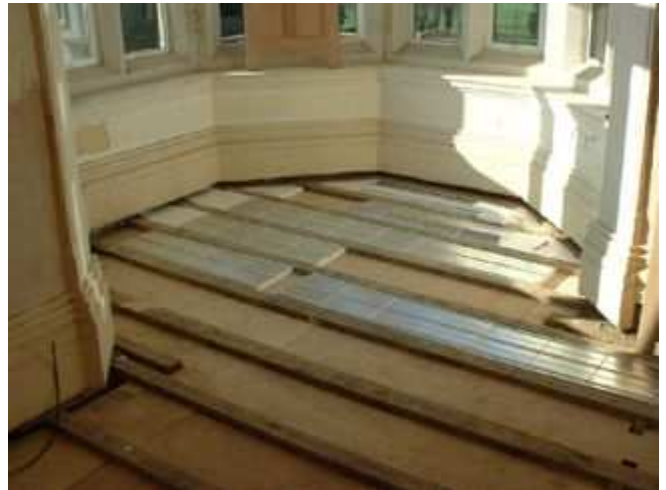
Existing joists batted and lined with ply 30mm below top of joist. IDEAL panels cut to fit tightly between.
