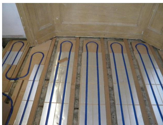
Rear Examples of IDEAL EPS (left) and IDEAL ECO (right) installed within existing joists.
