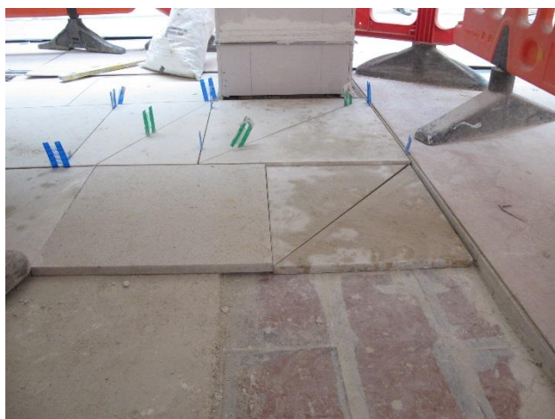
Final stone floor being installed directly on Screed Replacement Tile at New Bodleian Library, Oxford.
