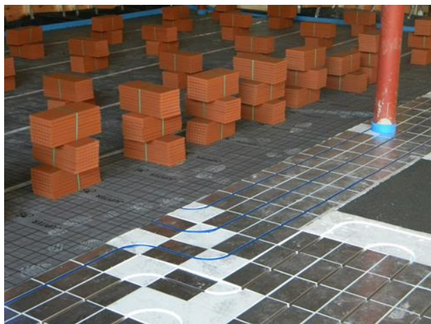
Photo showing Screed Replacement Tile being prepared for installation over underfloor heating system.
