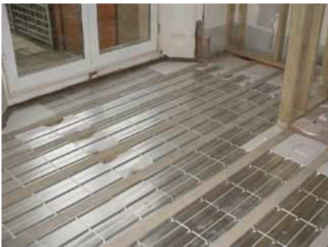
Jupiter Edge Zone (EZ) panels used to provide 3 pipes per joist void.
