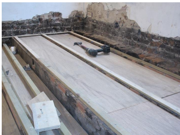
Detail showing ply installed between joists of Grade 1 listed building. Joists made level with timber furrings
