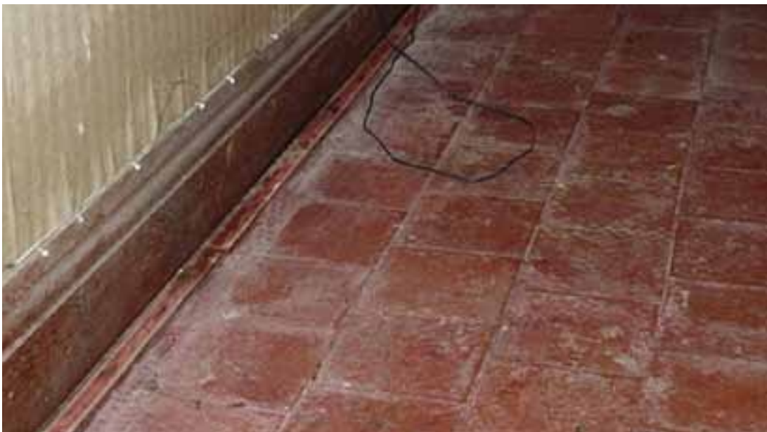
04 Salts appearing on the surface of a solid floor that has been very damp © Janice Gooch
