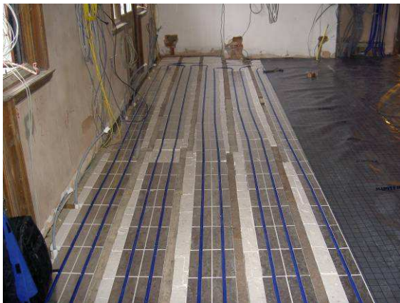
IDEAL System installed within existing joists. Resting on additional insulation resting on battens and ply supporting sheets.
