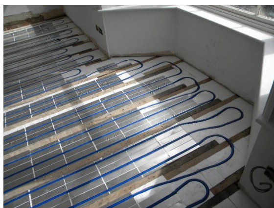
Rear Examples of IDEAL EPS (left) and IDEAL ECO (right) installed within existing joists.
