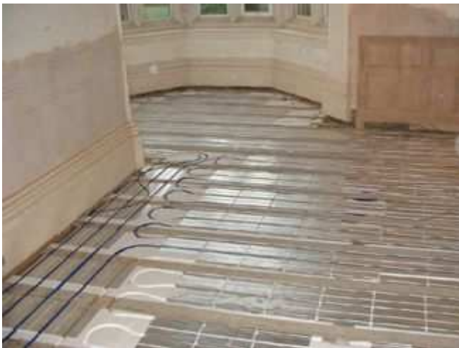
Flow and return pipes as well as circuit pipes channelled through joists.
