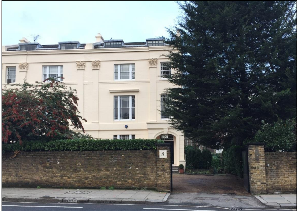
Photograph 2.1 (above): No. 8 Prince Albert Road, Front Façade.
