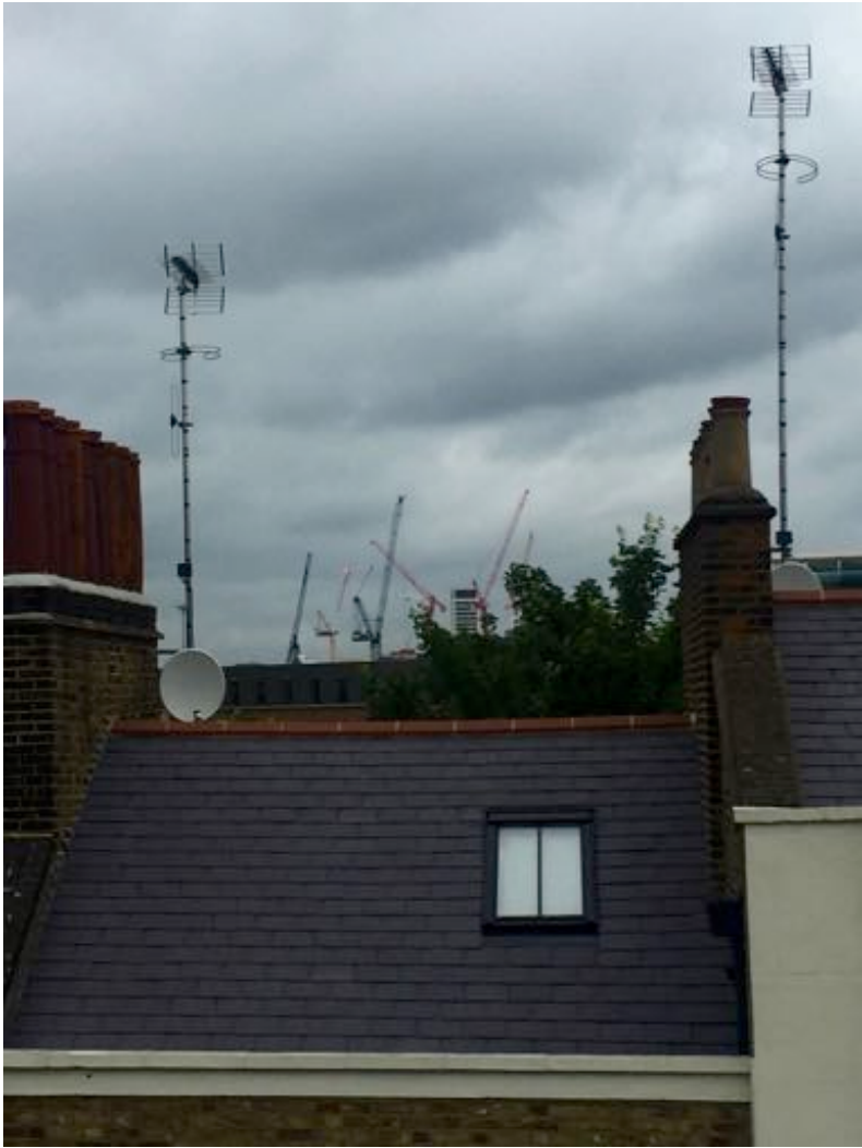
EXAMPLE OF IRS INSTALLATION (SATELLITE DISH, TV & RADIO AERIALS) (at 54 FREDERICK STREET)
