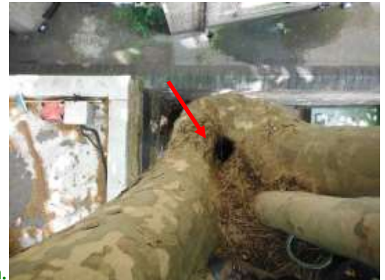
Looking down at the cavity entrance at 9m.
