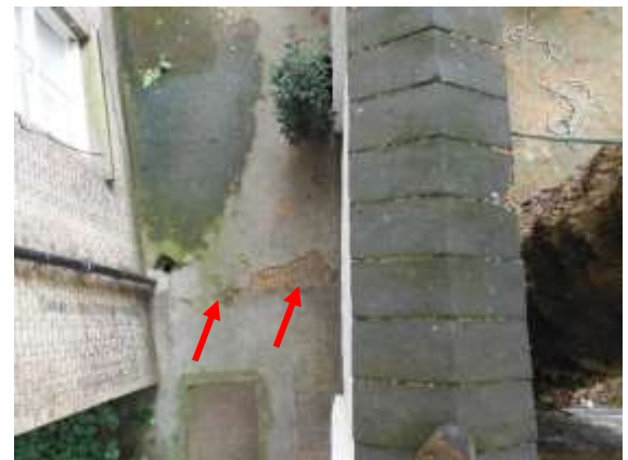
Looking down and slightly east at either side of the Northern boundary wall
