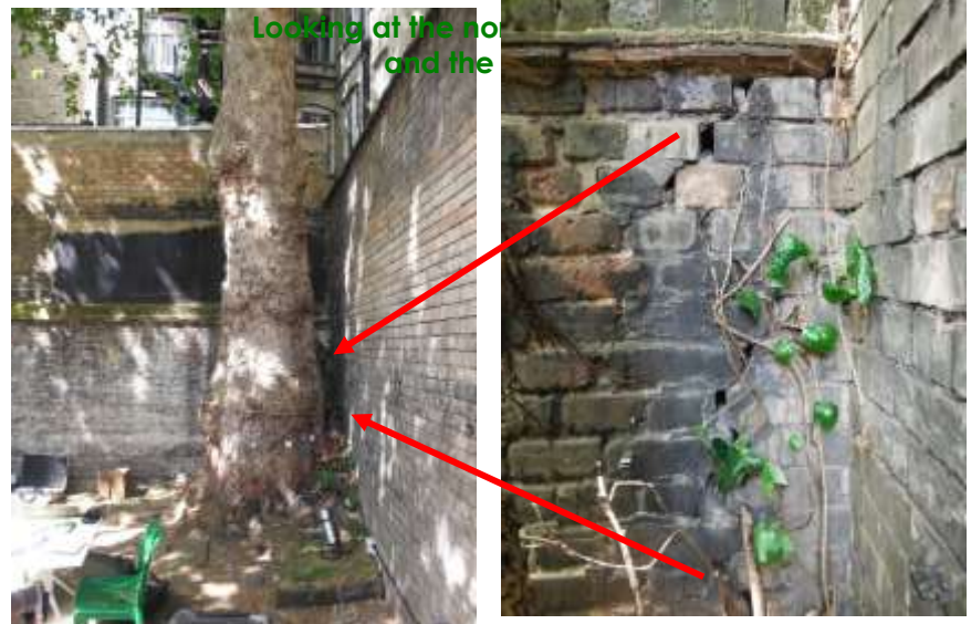
Looking west along the rear boundary wall.
