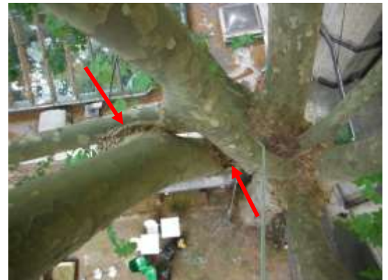
Looking west and downwards at the main canopy attachment.
