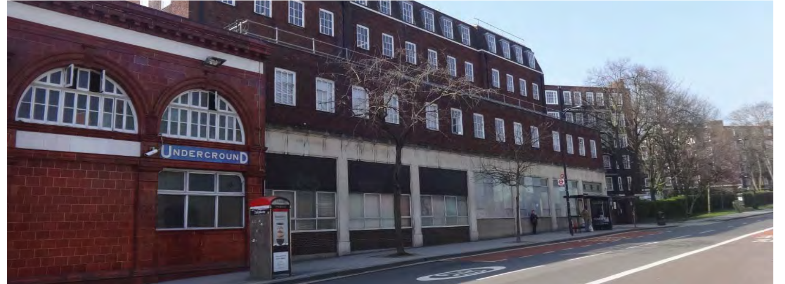
View of existing site and Chalk Farm Underground Station from Haverstock Hill
