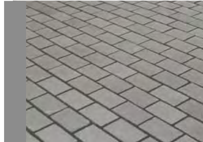
Granite sett paving
