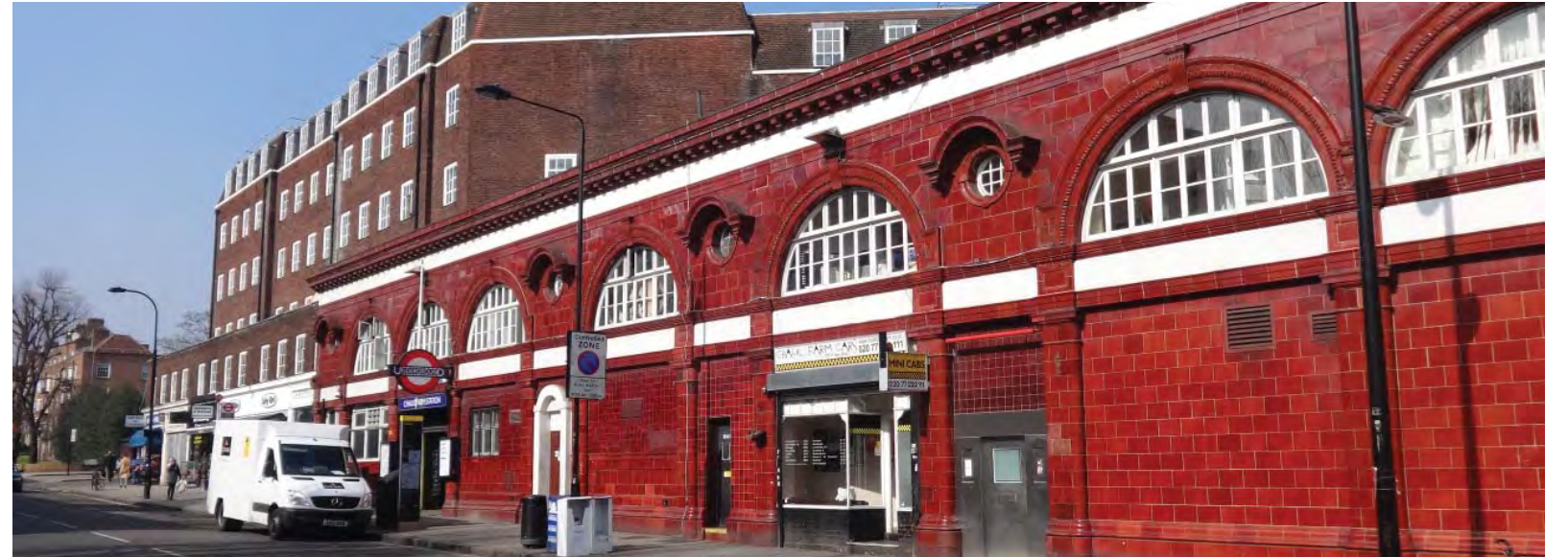
View of existing site and Chalk Farm Underground Station from Adelaide Road
