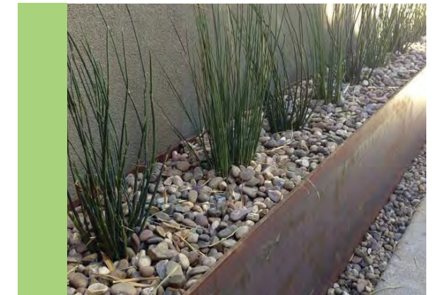
5mm thick 250 high metal retaining edge
