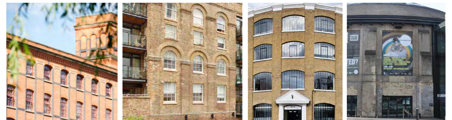
Camden Industrial Brickwork
