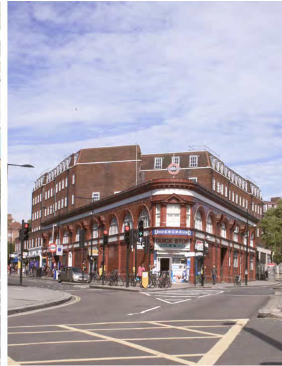
Key view from Chalk Farm Road of the station and site
