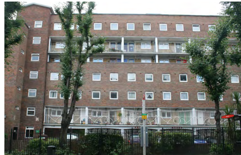
IV: Bridge House, Adelaide Road
