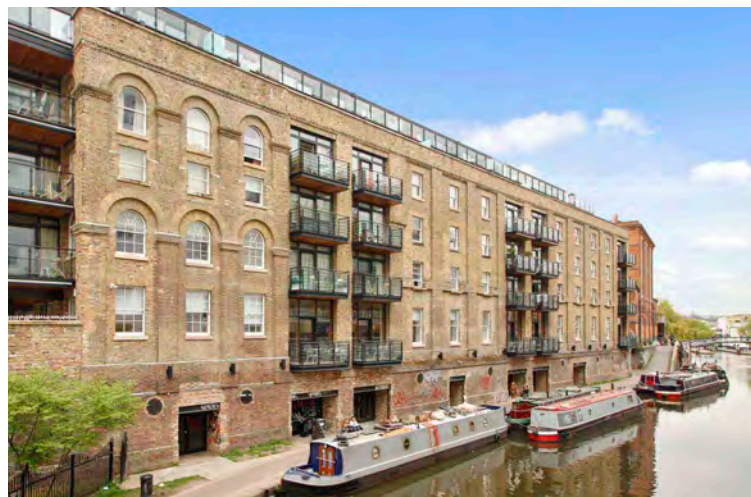
C: The Henson Building, Oval Road, Camden
