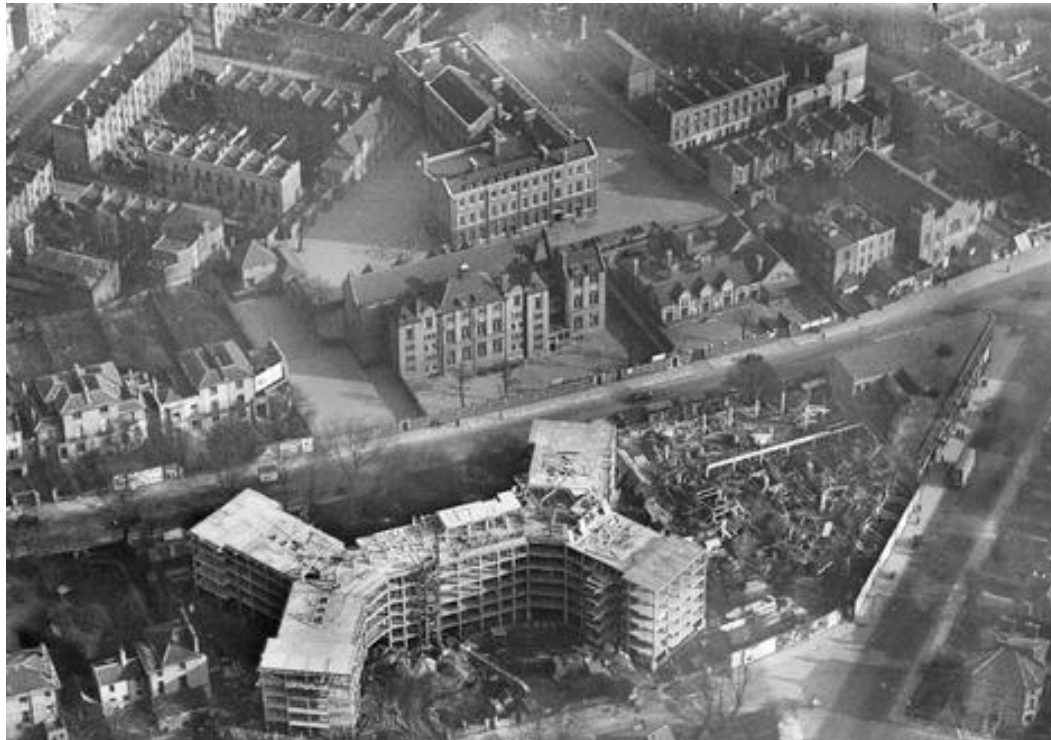
Eton Garage and Eton Place under construction
