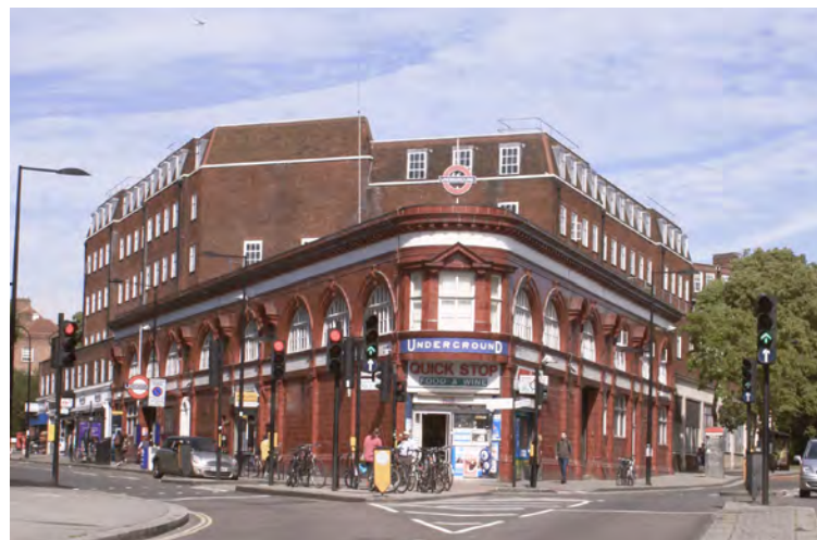
Chalk Farm Station: View from Chalk Farm Road
