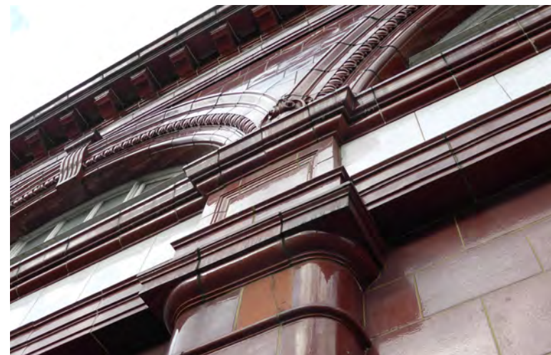
Chalk Farm Station: Detail of Faience Blocks
