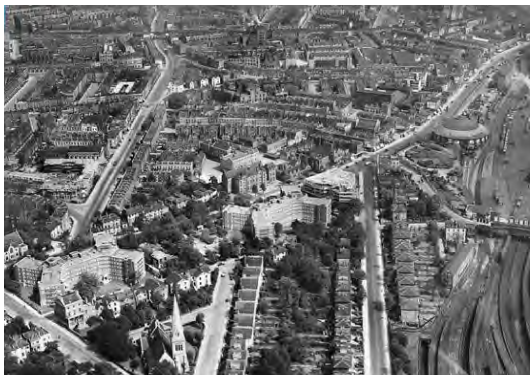
View from the North West with St Saviour's Church Spire in the foreground and the Roundhouse to the right
