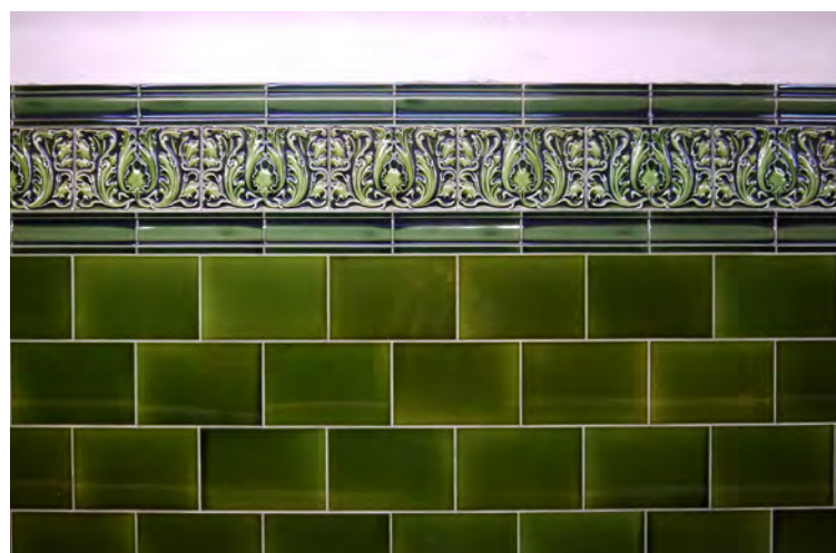
Chalk Farm Station: Interior tiling detail
